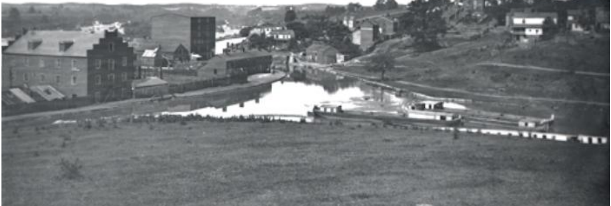
(Figure 18.) This 1865 photograph shows the extent of Harvie's Pond, which was fed by springs and creeks filling the natural ravine that separates Oregon Hill from Gamble's Hill. Evidence indicates that the tow path on the site of Venture Richmond's proposed amphitheater was originally a "substantial embankment" 30 feet wide to hold back this volume of water. (Source: Library Company of Philadelphia)
