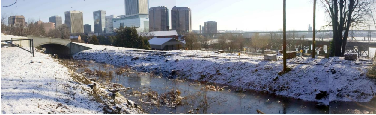
(Figure 46.) The railroad tracks connecting the iron works on Belle Isle with Tredegar are seen here on the top of the tow path. Venture Richmond has proposed removing these railroad tracks, which only add a few inches to the height of the towpath, in order to improve the sight lines of the amphitheater and to build a bike path. Venture Richmond successfully opposed putting a dedicated bike lane on the new 2 nd Street connector, so replacing the authentic Tredegar-Belle Isle rail link with a bike path would be a 100 foot bike trail to nowhere.
