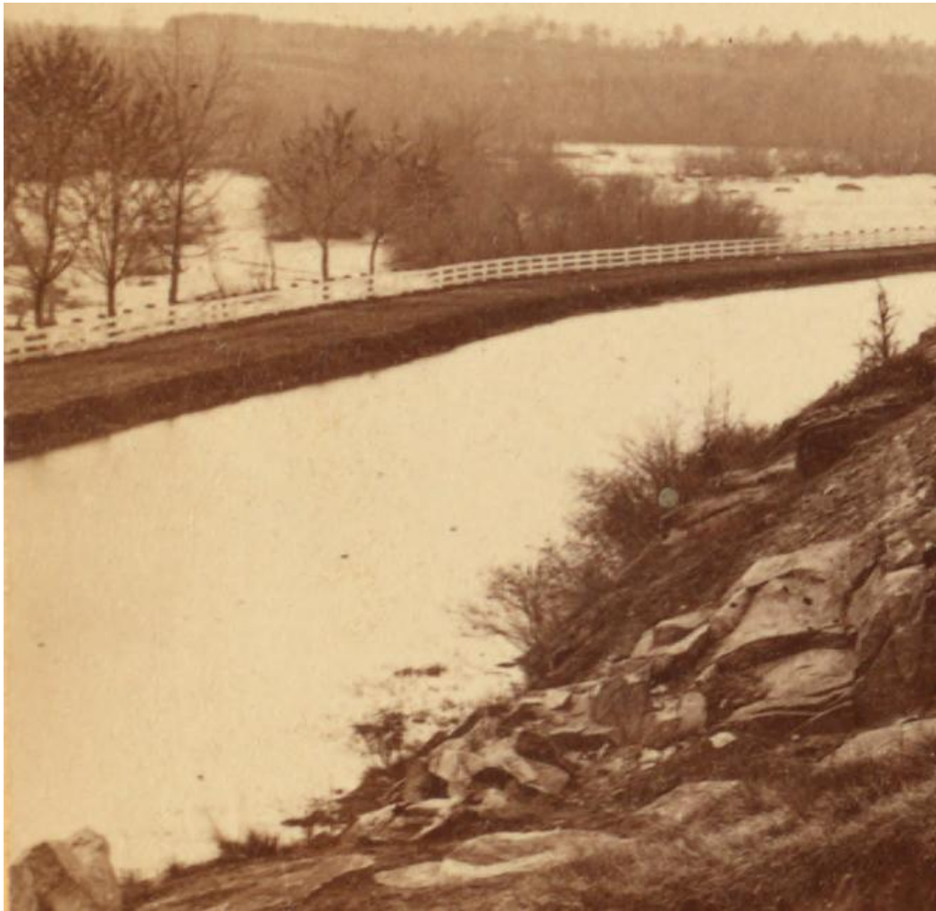
(Figure 27.) “Looking up the River at Hollywood Cemetery,” (detail) David H. Anderson, Civil War era (Source: New York Public Library) The water level is at least two feet below the top of the tow path in this photograph of the canal looking west from Hollywood Cemetery. Venture Richmond’s consultant has inaccurately stated that there was limited clearance between the tow path and the water level in the canal.
