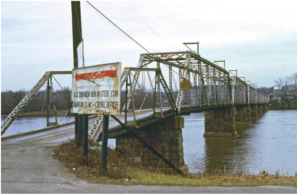
(Figure 47.) The stone pylons in the James River and a bridge section on the banks of Belle Isle have survived from this bridge, which was photographed around 1972. A former bridge on these same pylons carried the Tredegar Branch of the Richmond and Danville Railroad, connecting Tredegar Iron Works with Old Dominion Iron and Nail Company on Belle Isle. (Source: VintageRVA.blogspot.com )
