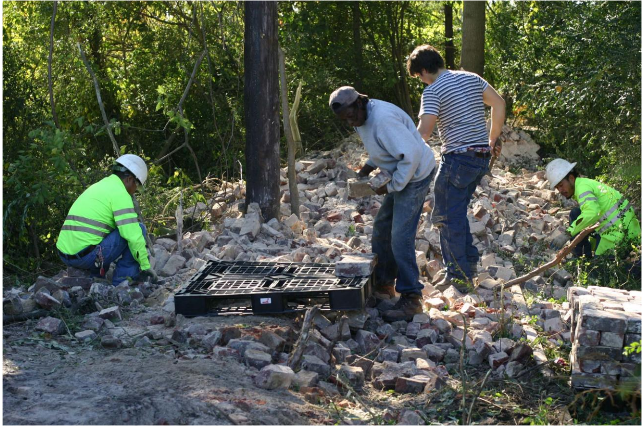
(Figure 51.) A bulldozer accessed the 100 foot long Tredegar wall on city property through Venture Richmond property. This contractor was not hired as part of the construction of the 2 nd Street Connector. Contractors were photographed at the scene of the illegal demolition stacking the bricks on pallets within an hour of the demolition. No entity has been held accountable for hiring the contractor to demolish the Tredegar wall on City of Richmond property without a permit. Was the removal of this wall anticipatory demolition?
