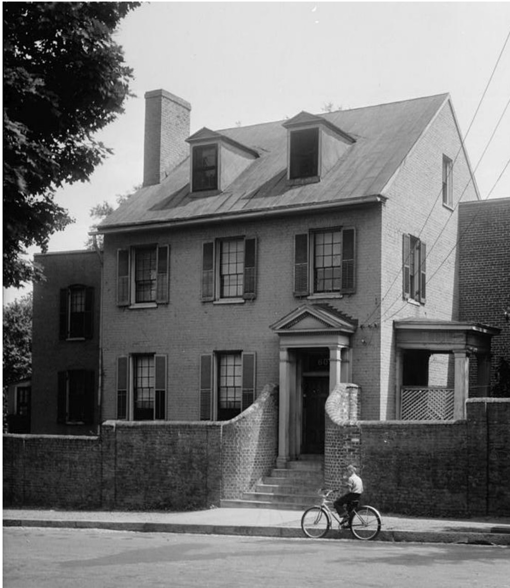
(Figure 53.) The Samuel Parsons House, 601 Spring Street, Historic American Buildings Survey, c. 1933, 44-RICH, 78—1 (Source: Library of Congress) Samuel P. Parsons served as the Superintendent of the Canal in 1840 when the canal was expanded to Lynchburg. The Parsons House is a contributing structure to the Oregon Hill Historic District, and the park across Spring Street from the house is named for Parsons. (Source: Library of Congress)
