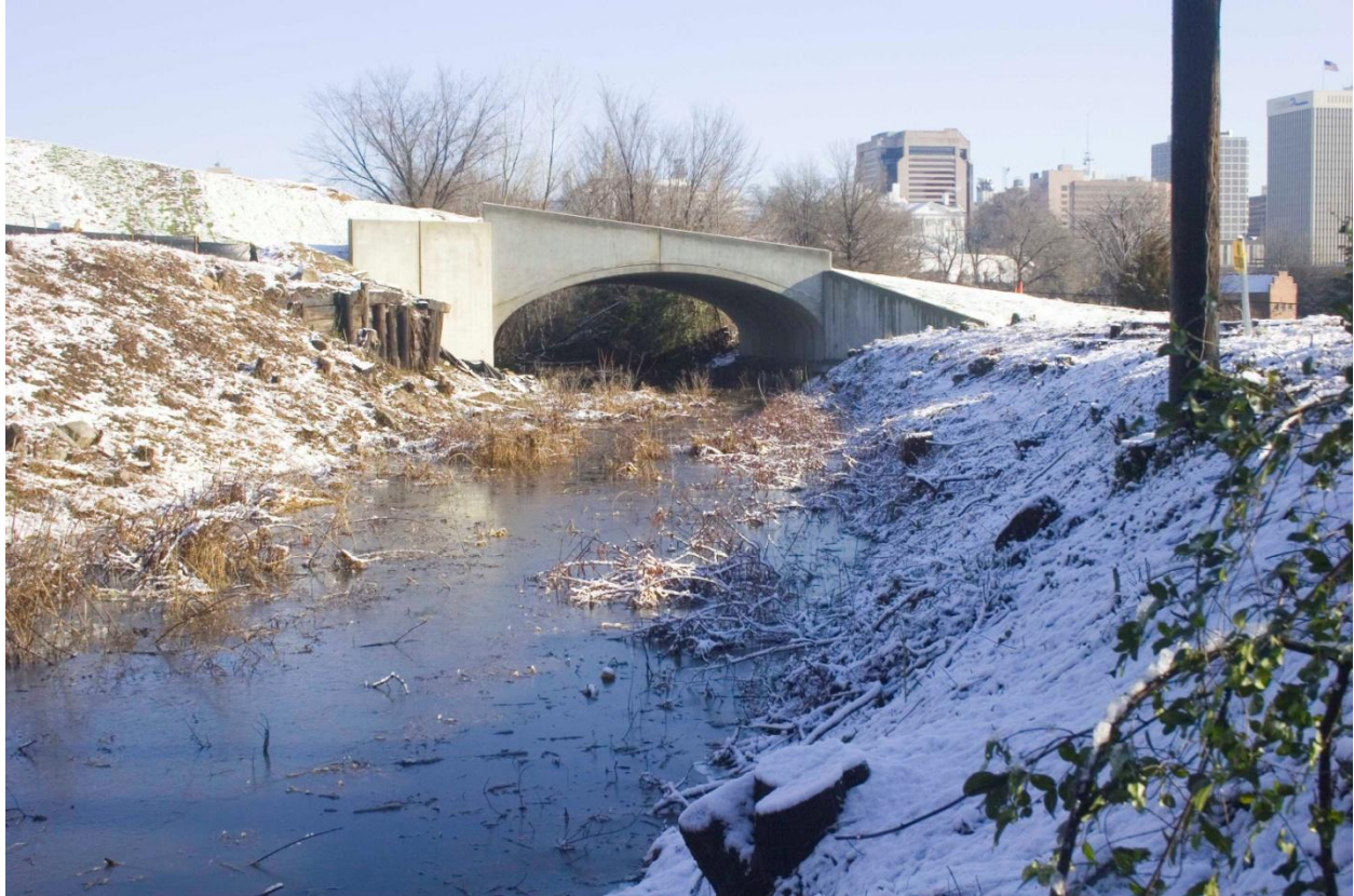
(Figure 12.) In 2012, the Richmond City Council approved the expenditure of $385,000 to protect the canal by constructing this bridge over the canal as part of the construction of the 2 nd Street Connector.
