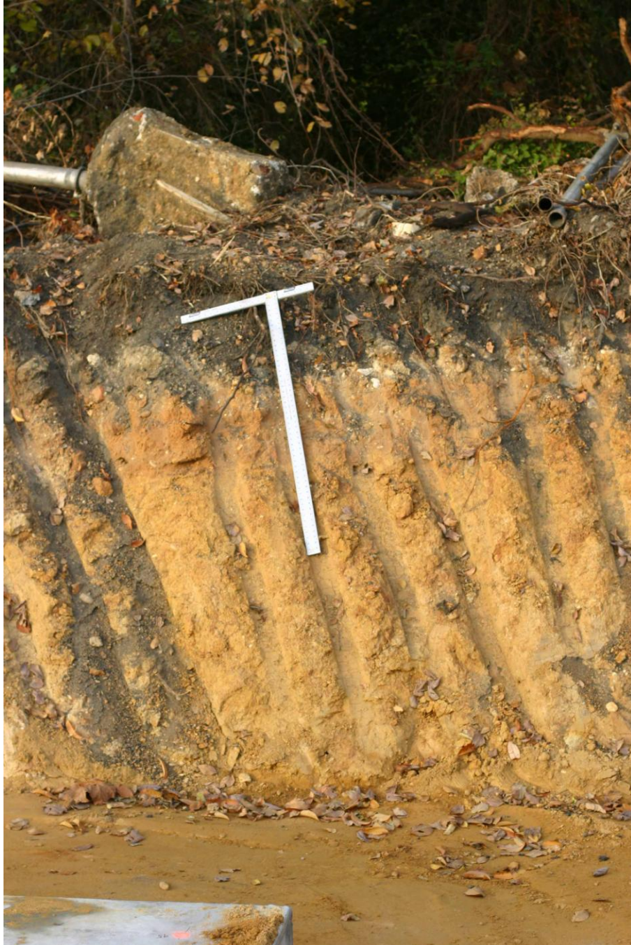
(Figure 34.) The James River and Kanawha Canal was a carefully engineered structure, designed to withstand the vicissitudes of weather and traffic, while holding back the considerable volume of water in the canal. This cross section of the canal was revealed when the 2 nd Street Connector was constructed in 2012. This cross section exposes the layer of clay that was “puddled” in a process to make an impermeable water-tight canal bank.
