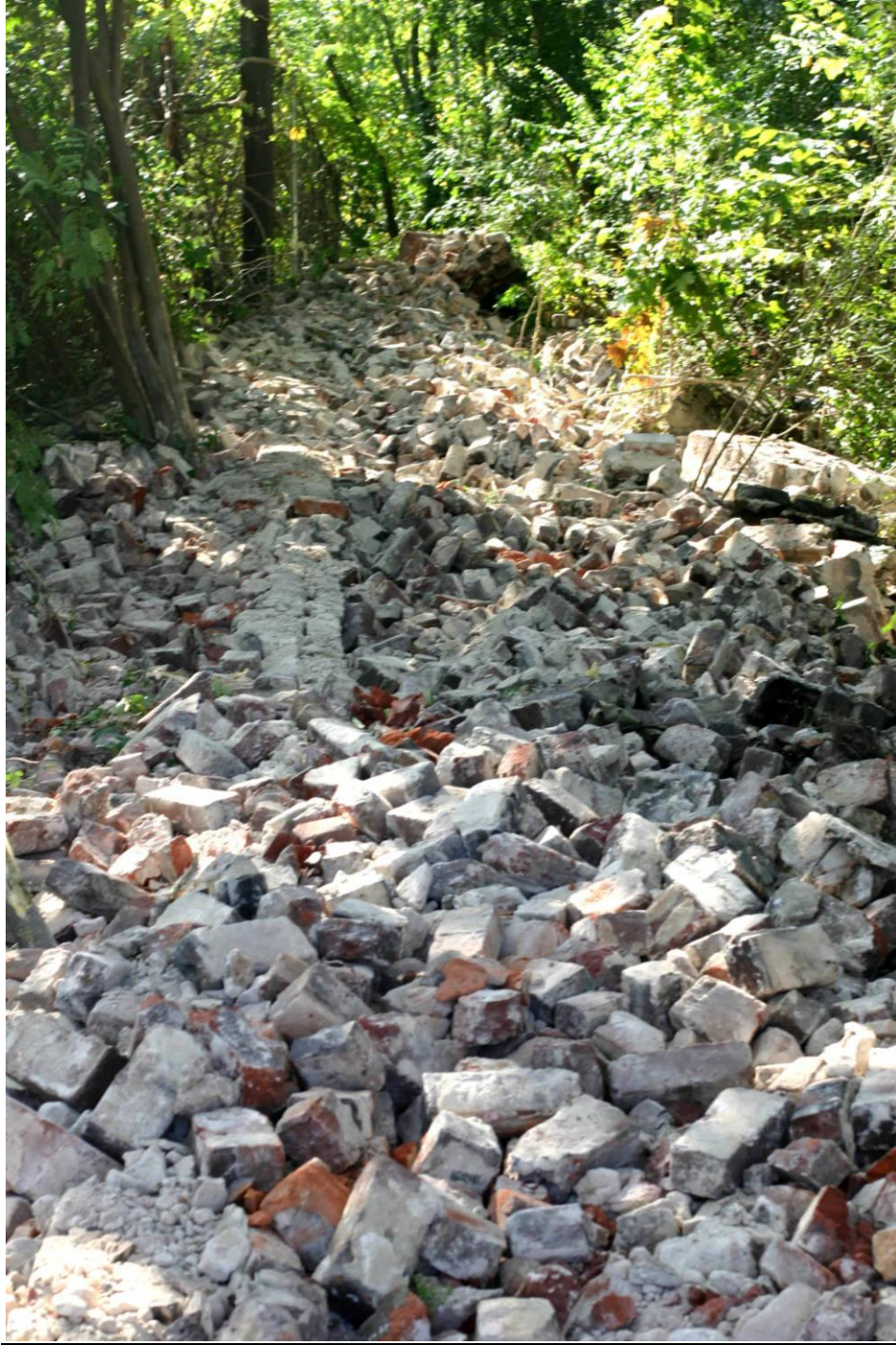
(Figure 50.) On October 16, 2012 the historic eight foot tall Tredegar wall was illegally demolished by a bulldozer on City of Richmond property on the site of Venture Richmond’s proposed amphitheater. Was this wall removed as anticipatory demolition before the regulatory review of Venture Richmond’s proposed amphitheater, which now includes this City of Richmond property?
