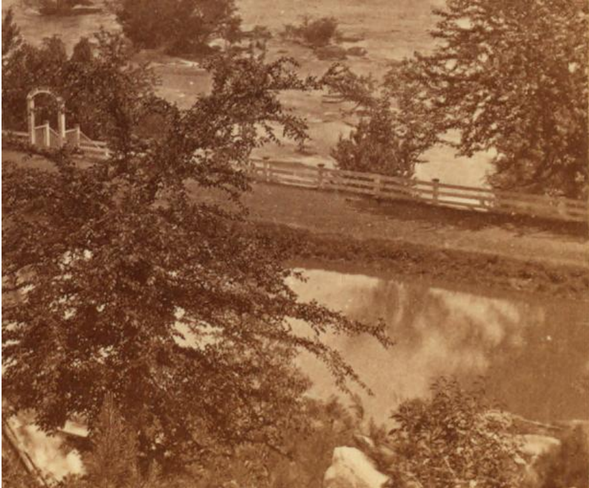
(Figure 28.) Canal from Hollywood Cemetery (detail), Civil War era. The canal at Hollywood Cemetery provided a picturesque setting that was often photographed. These photographs now provide useful information in determining the elevation of the tow path above the water level of the canal. The tow path in this photograph was at least two feet above the water level of the canal. This provided a margin of safety during freshets that could cause flooding and expensive damage the canal banks. Flooding was historically the cause of the most serious damage to the canal. (Source: New York Public Library)
