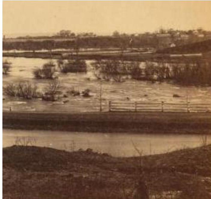
(Figure 26.) Canal with Belle Isle in background (detail). The tow path is at least two feet above the water level of the canal in this Civil War era photograph. The fence on the tow path provides a convenient bench-mark to gauge the tow path's elevation above the water level. (Source: New York Public Library)
