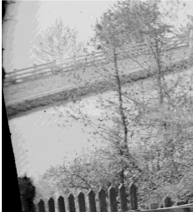
(Figure 25.) "Richmond Va. View from Hollywood Cemetery," (detail) John Keekie, c. 1865 LC-B811-929 (Source: Library of Congress). Note the tow path in this Civil War era photograph is at least two feet above the water level in the canal based on the adjacent fence for comparison.
