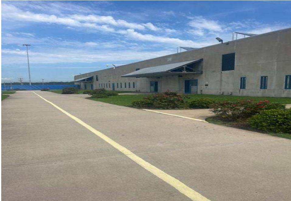
Housing Unit Exterior
