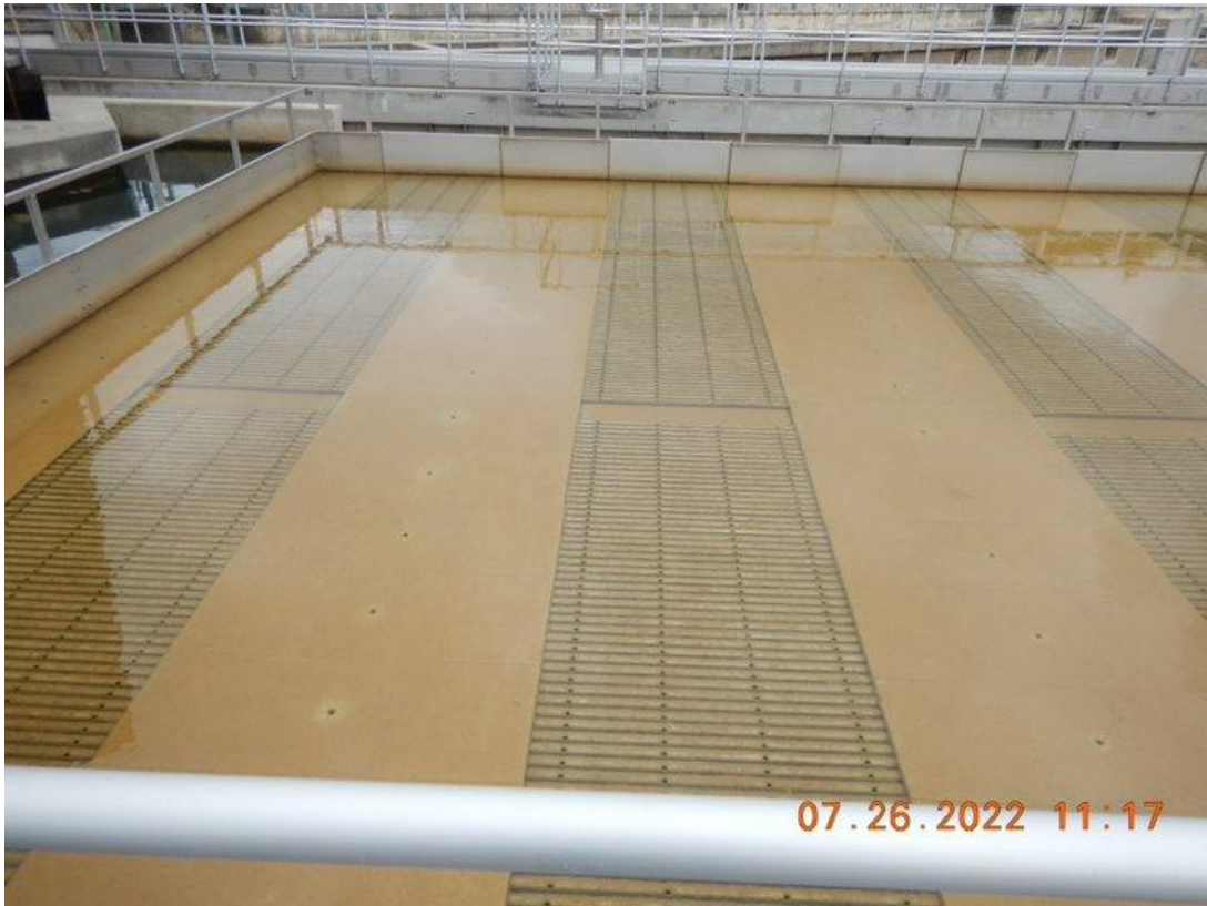
Photograph 22. Plant 1 plate settlers.
