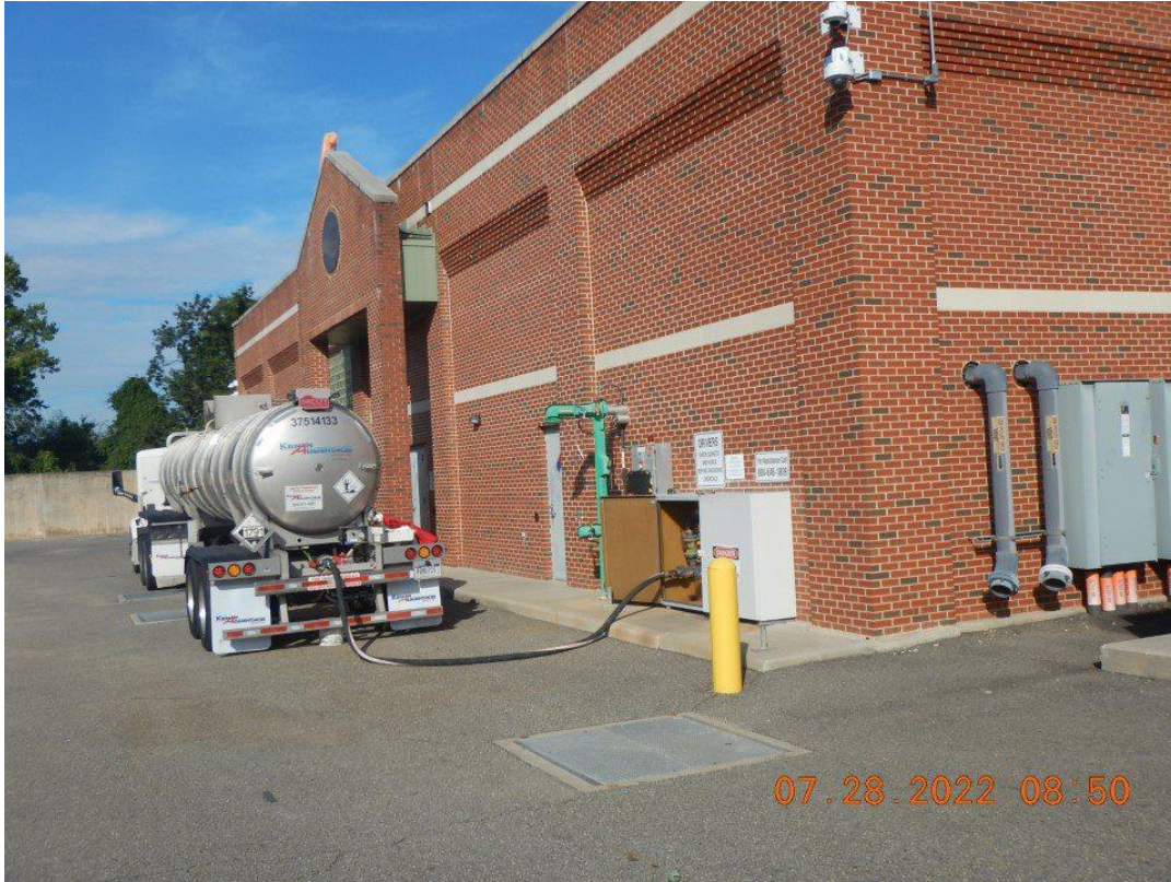
Photograph 121. Sodium hypochlorite offloading in process at West Chemical Building.
