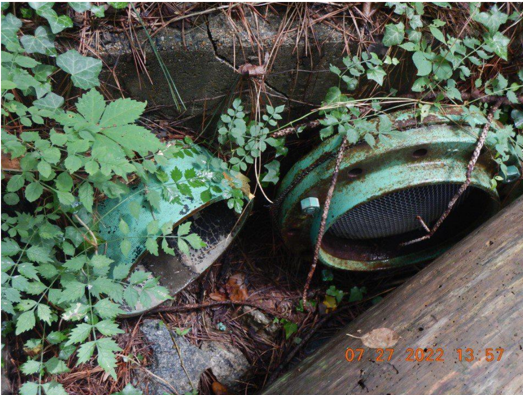
Photograph 90. Overflow and/or discharge pipes from the Huguenot Road Tank.
