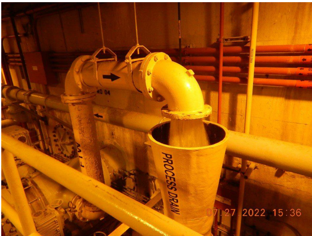
Photograph 111. Plant 1 pipe gallery and Filter 4 filter-to-waste drain in process.
