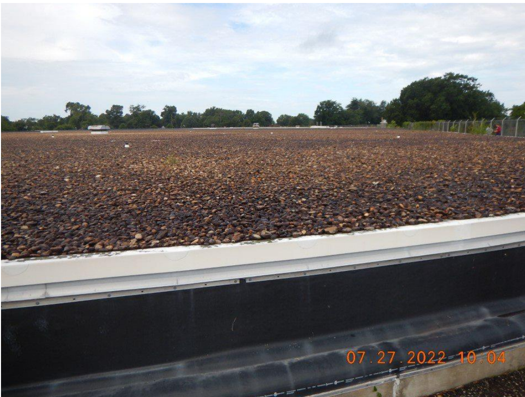
Photograph 54. Roof of Byrd Park Reservoir.
