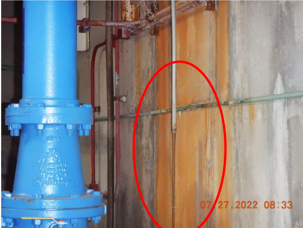
Photograph 43. Process water pipe discharging to floor on lower level of Korah 2 and 3 Pump Station
