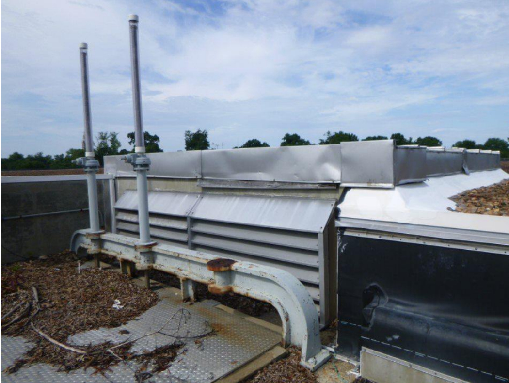
Photograph 65. Vents on eastern side of north walkway at Byrd Park Reservoir.
