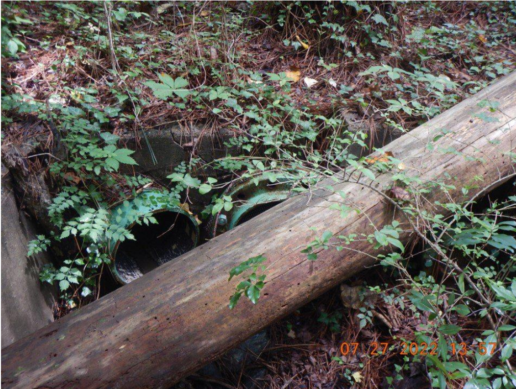
Photograph 89. Overflow and/or discharge pipes from the Huguenot Road Tank.
