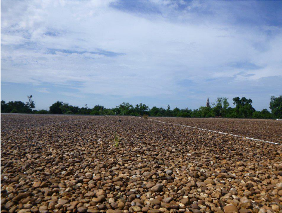
Photograph 53. Roof of Byrd Park Reservoir.
