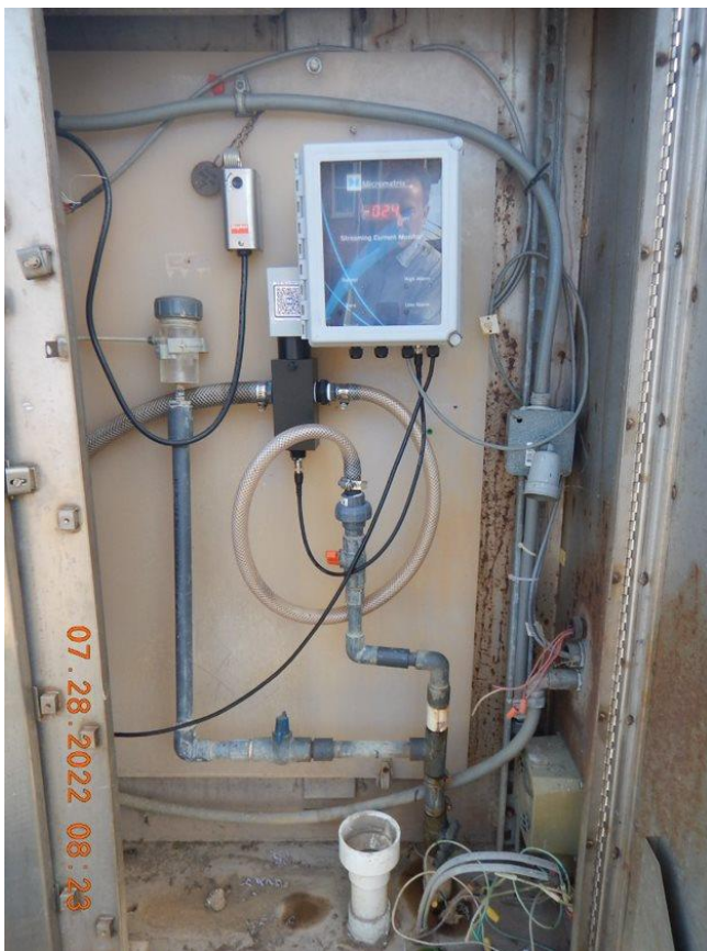
Photograph 117. Streaming current monitor for Plant 1, reading -0.24 mV.
