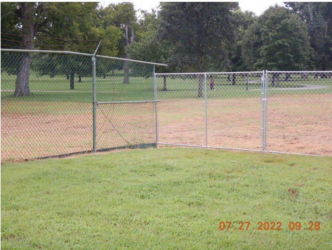
Photograph 50. Fencing at the Trafford Pump Station.
