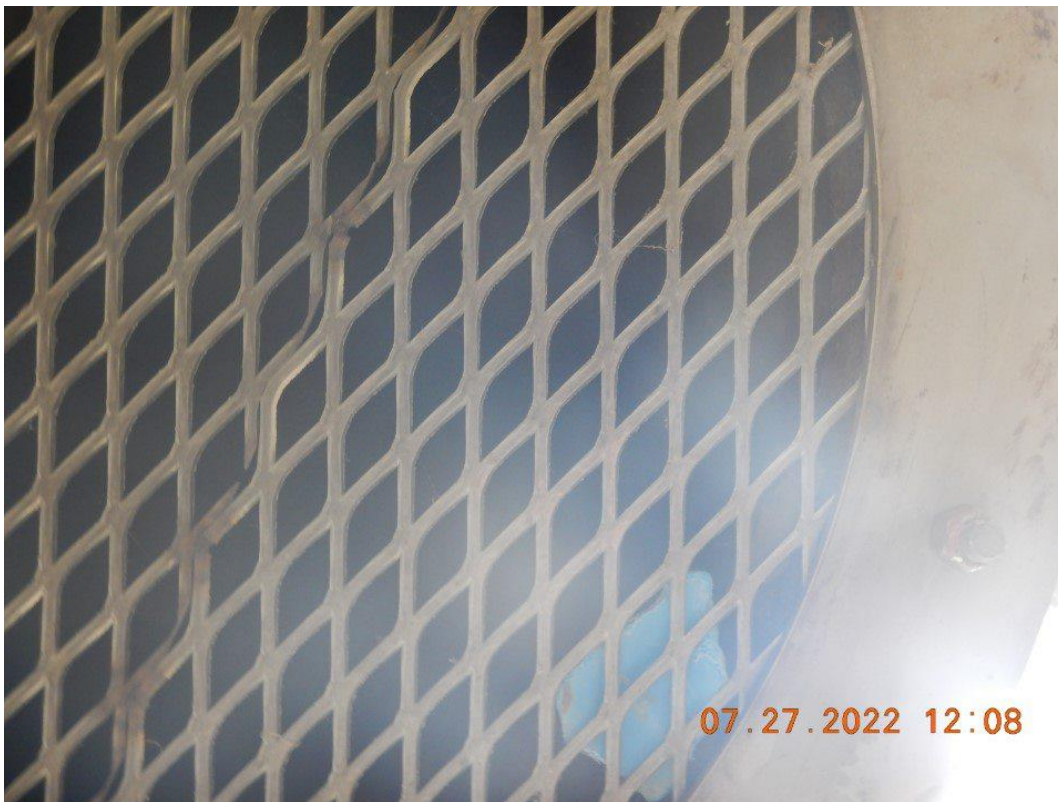
Photograph 78. Rough mesh on overflow at Jahnke Road Tank.
