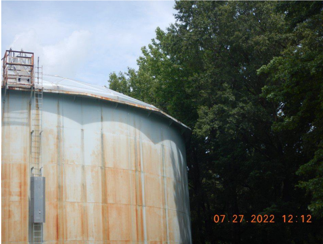
Photograph 75. Overhanging trees at rear of Jahnke Road Tank.
