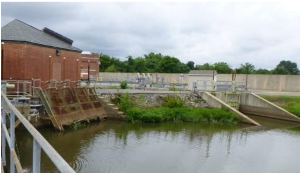
Photograph 10. Raw water intake and out of service screens.
