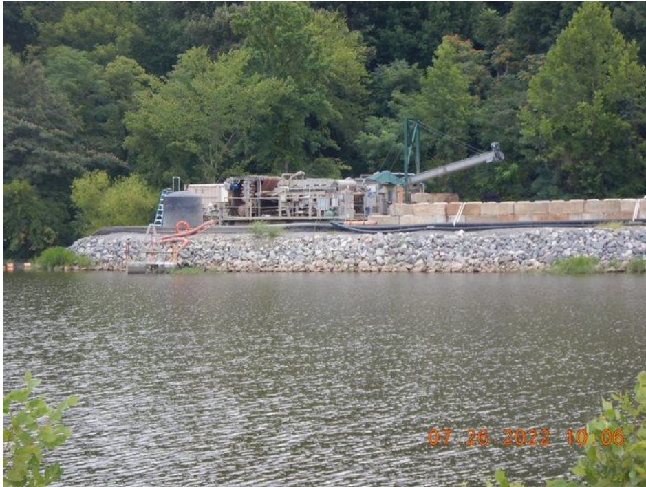
Photograph 3. Lagoon waste processing and dewatering operation.
