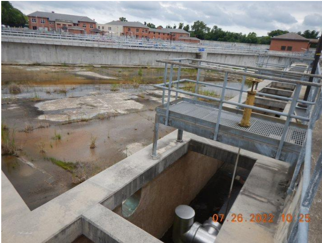
Photograph 9. Inactive basin, former sedimentation basin area.
