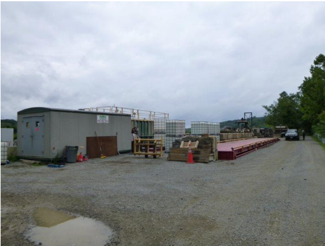
Photograph 6. Polymer containers without secondary containment in the dewatering area.
