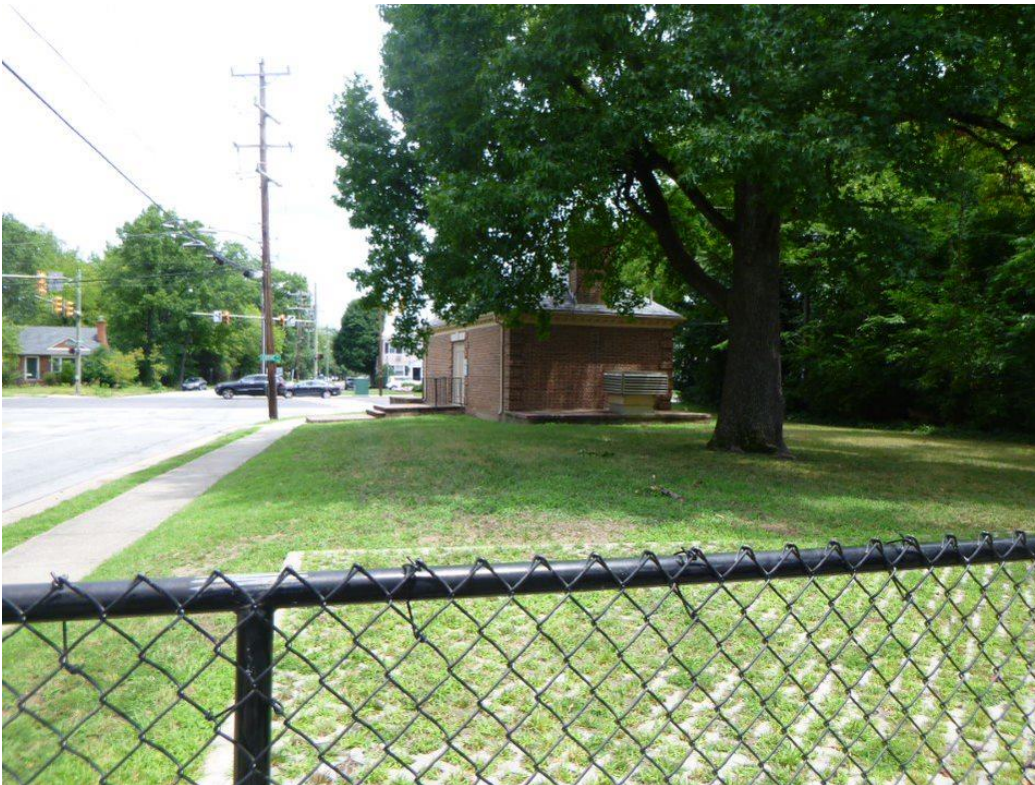
Photograph 108. Four-foot fencing at Westhampton Pump Station in highly trafficked residential area.
