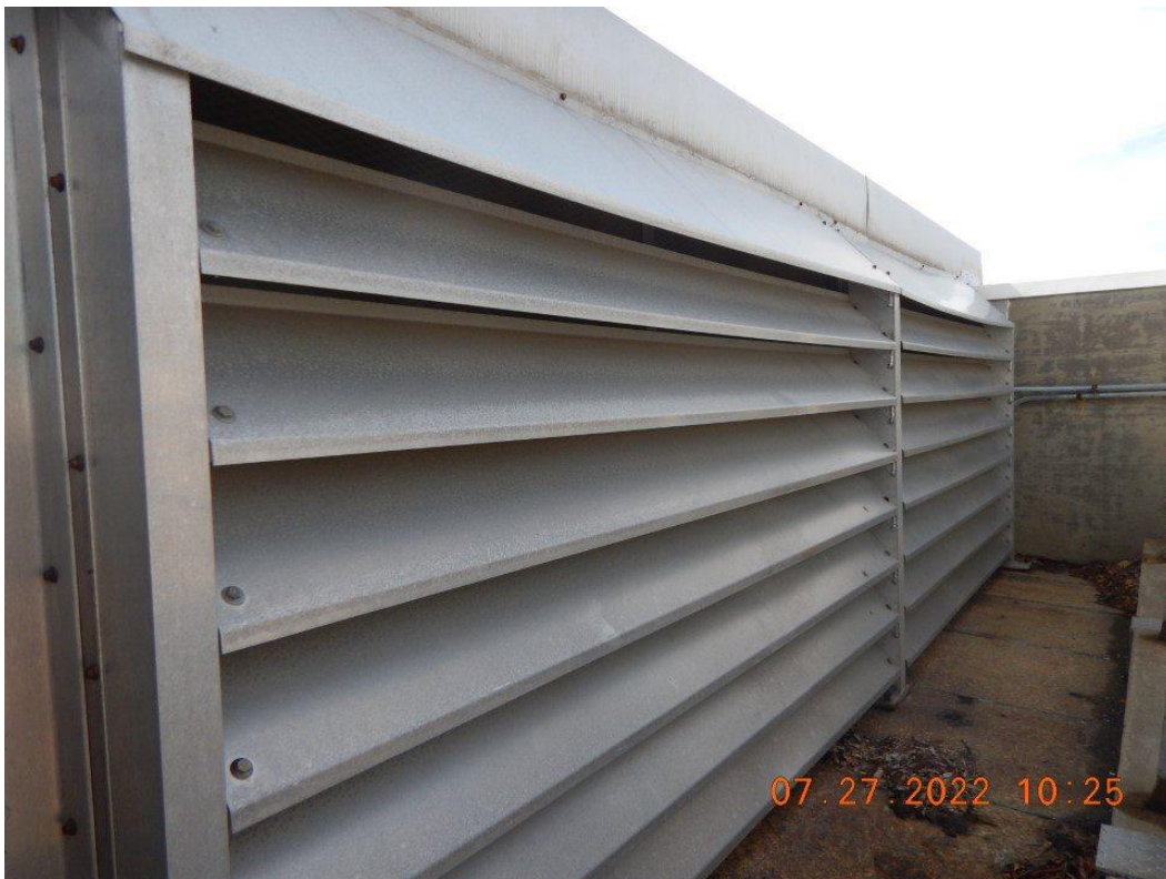
Photograph 64. Vents on western side of north walkway at Byrd Park Reservoir.
