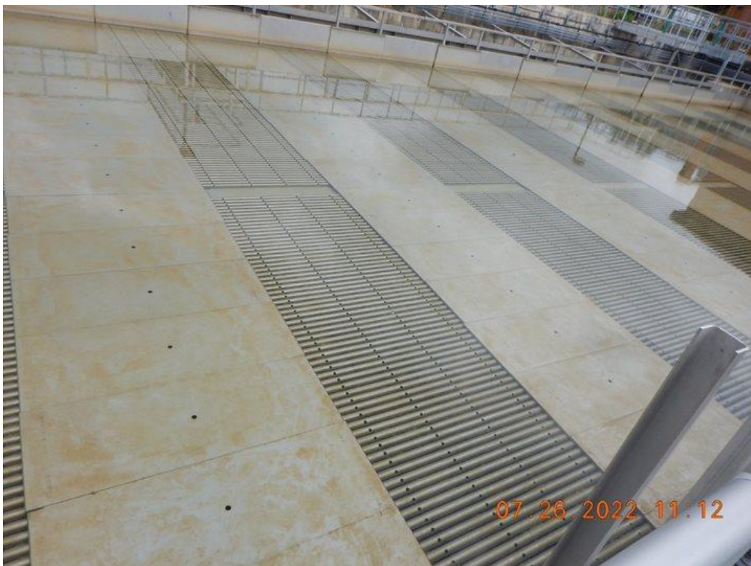
Photograph 23. Plant 2 plate settlers.
