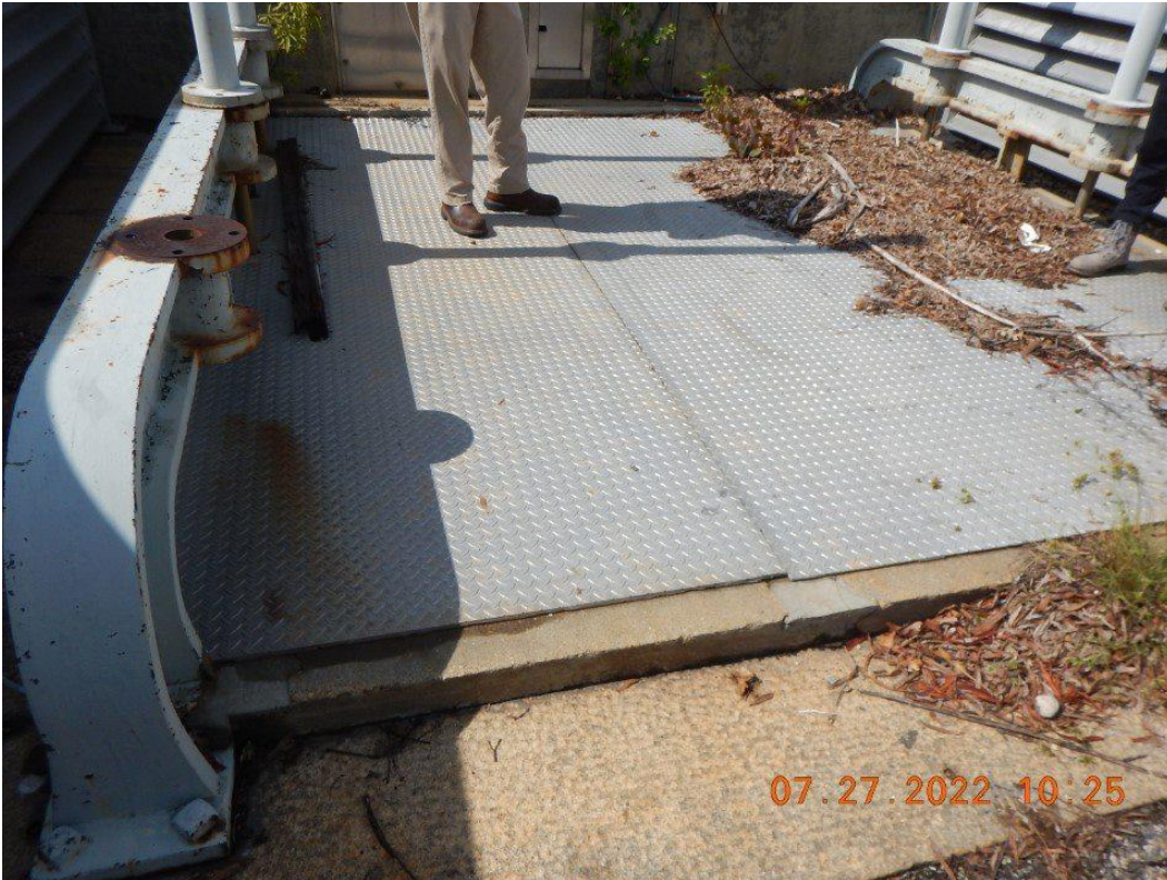
Photograph 66. Metal plates in between vents in access area on northern walkway of Byrd Park Reservoir.
