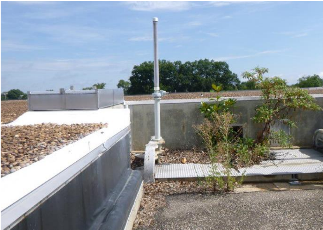
Photograph 68. Southern access walkway at Byrd Park Reservoir.
