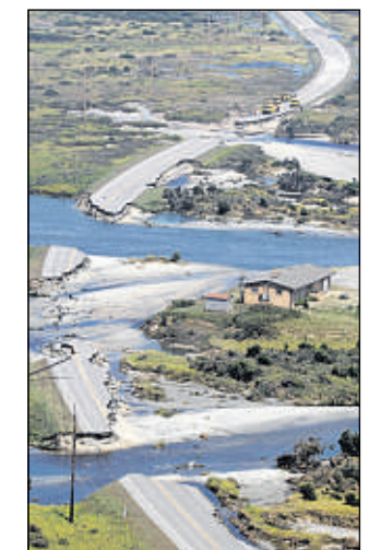
2011, THE ASSOCIATED PRESS Route 12 on Hatteras Island was cut in five places after Hurricane Irene hit the area.
