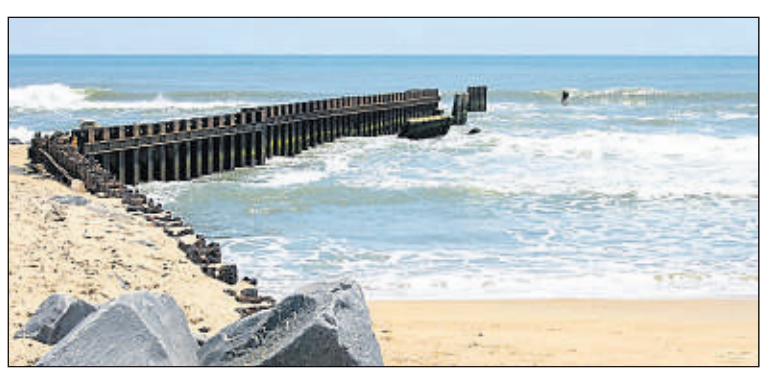
KIRA RIDER/TIMES-DISPATCH A seawall was built on Hatteras Island to help prevent erosion.
