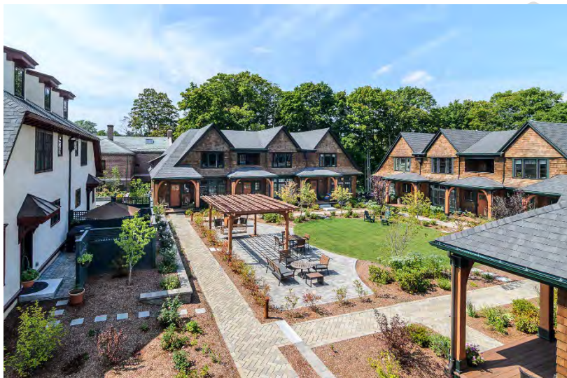
Example of housing units facing a courtyard.
