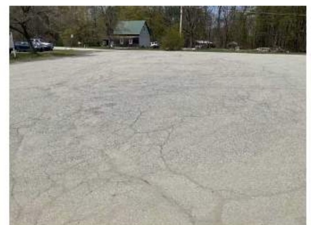
54 - PARKING LOT ASPHALT, MILL & OVERLAY
