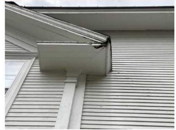
8 - ROOF EDGE CONDITIONS DETAIL
