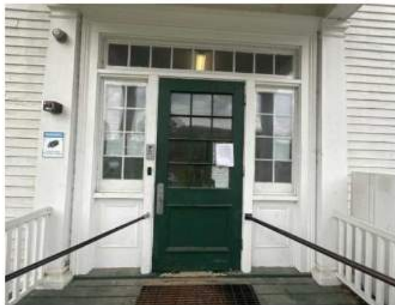
6 - MAIN BUILDING ENTRANCE
