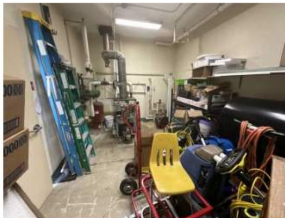
24 - 95' ADDITION BOILER ROOM
