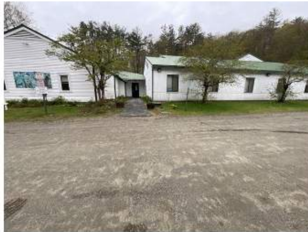
1 - OVERVIEW OF ACCESSIBLE PARKING AREA
