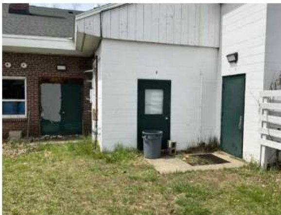
5 - EXTERIOR STEEL DOORS
