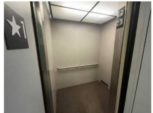
16 - CAB FINISHES OF ELEVATOR
