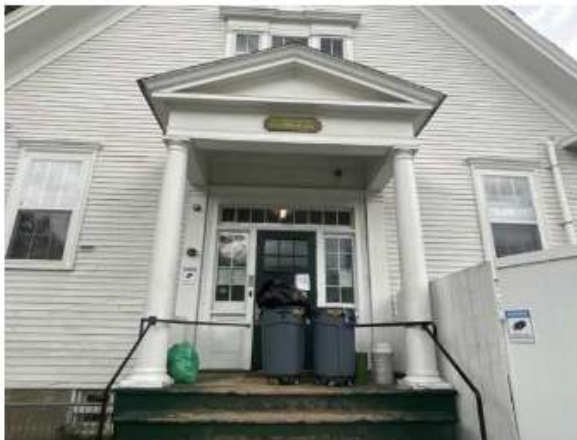
5 - FRONT FACADE PORTICO
