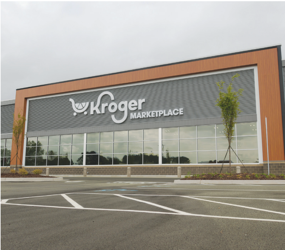
The newly constructed Kroger Marketplace building located at 2301 College Station Road in Athens, Georgia, on March 30, 2025. The new Kroger Marketplace is set to open in May 2025. PHOTO/KALEB TATUM
