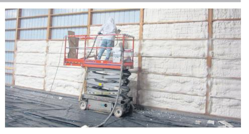
GreenTech Spray Foam Insulation saves businesses and homeowners an average of 40-60 percent on energy with their innovative foam. This insulation prevents excess moisture and air inside, adds structural support, lessens heating and cooling time, deters pests and decreases dust, noise and mold production.
