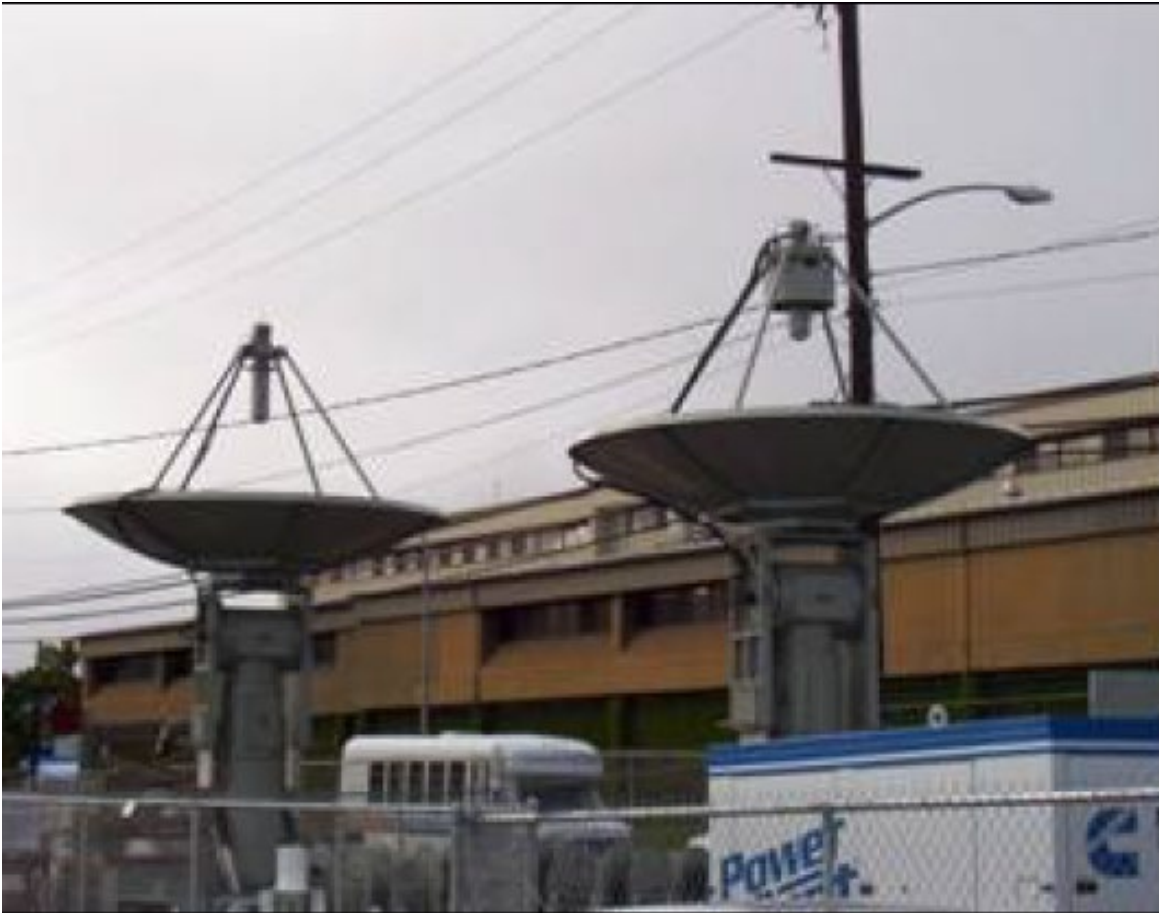
Figure D-3: Mobile Range Safety System Equipment
