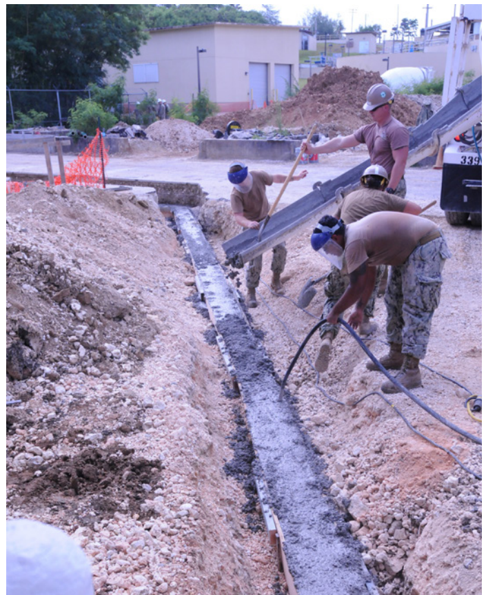
Naval Mobile Construction Battalion 1 Places Concrete at the NMCB 1 Fena Water Treatment Storage Building
