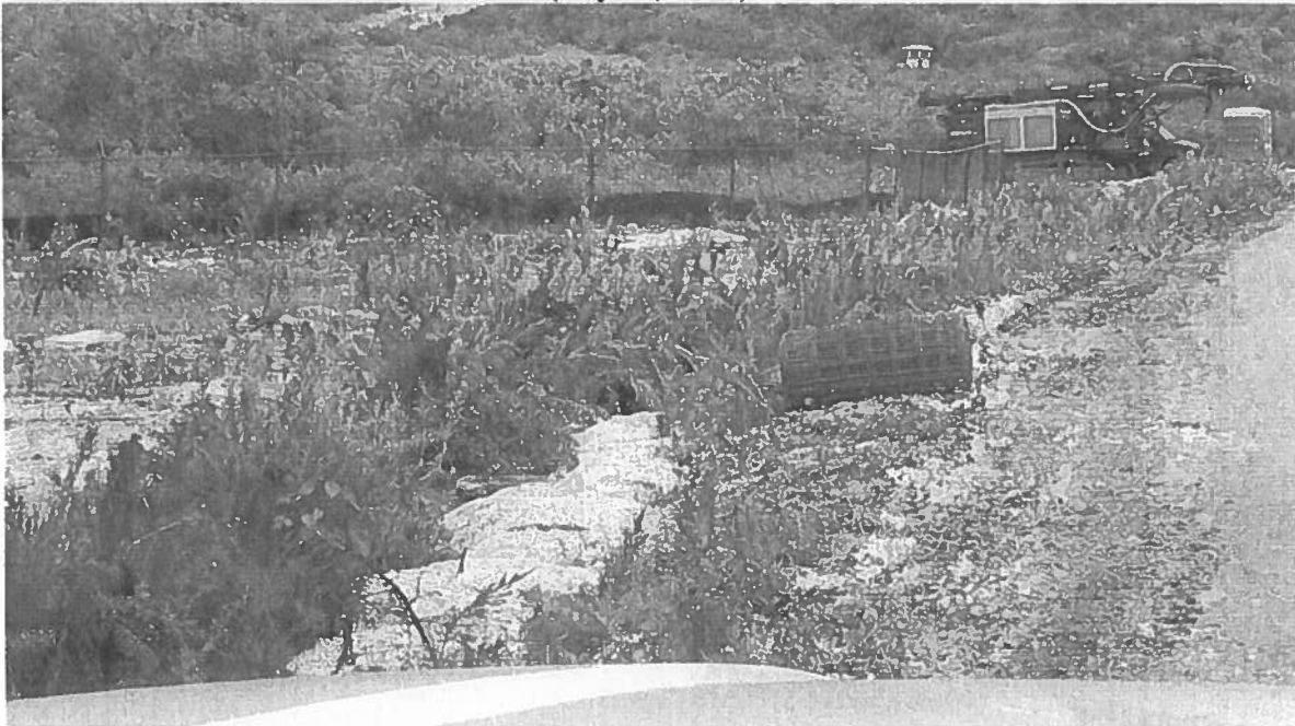
Perimeter berm which conveys runoff to Pond 3. Ironwood saplings and a large amount of accumulated sediment obstruct the flow. (July 23, 2021)
