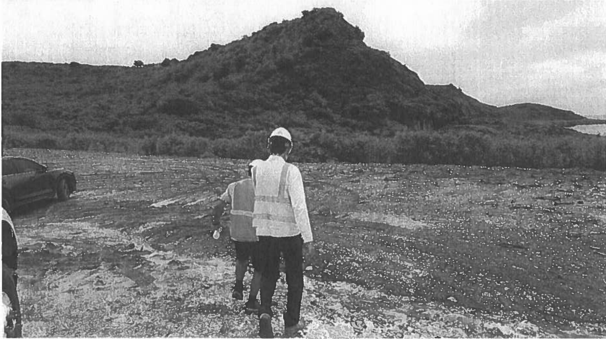
View looking from site office to area where start of Pond 4 berm and swale should be located. (July 23, 2021)
