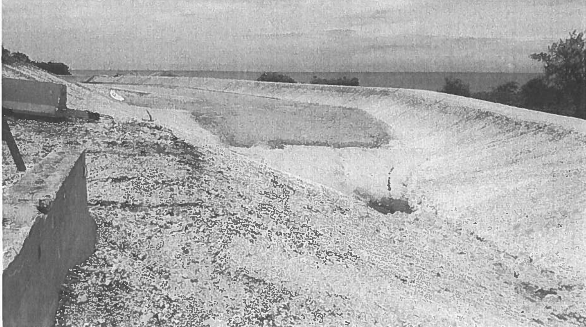
Pond 3. Overflow weir in distance is not yet finished – still requires stone riprap. (July 23, 2021)
