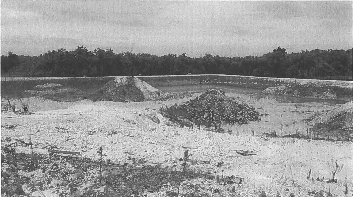
Pond 1. Note stockpiles of earth material, which reduce pond capacity. Also note high water mark from the previous storms. (July 23, 2021)
