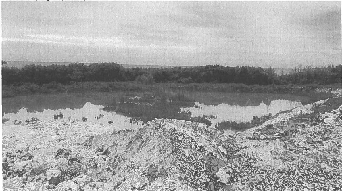
Pond 2, with accumulated runoff and sediment from storm. This pond does not appear to be finished. (July 23, 2021)
