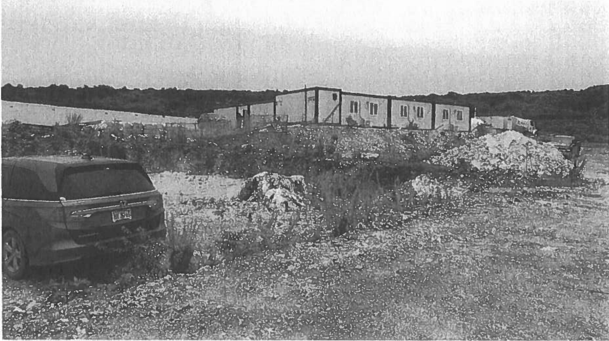
Looking back upslope toward Project Site Office, showing start of (revised) Pond 4 excavation (July 23, 2021)
