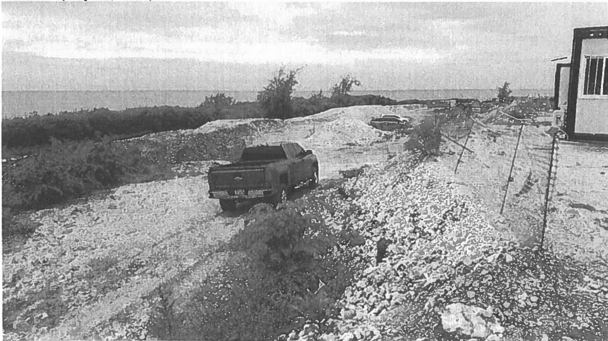
View looking downslope where Pond 4 berm construction has begun, and toward Pond 2 in distance. (July 23, 2021)
