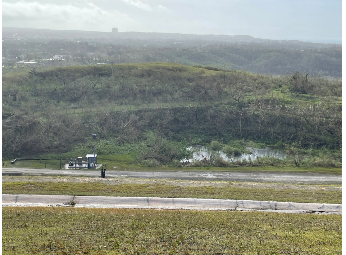
Figure 5. Photo of the Landfill Gas Flare and Pond 4 taken from the cap when staff made it back to the site after the storm on the 25 th of May.
