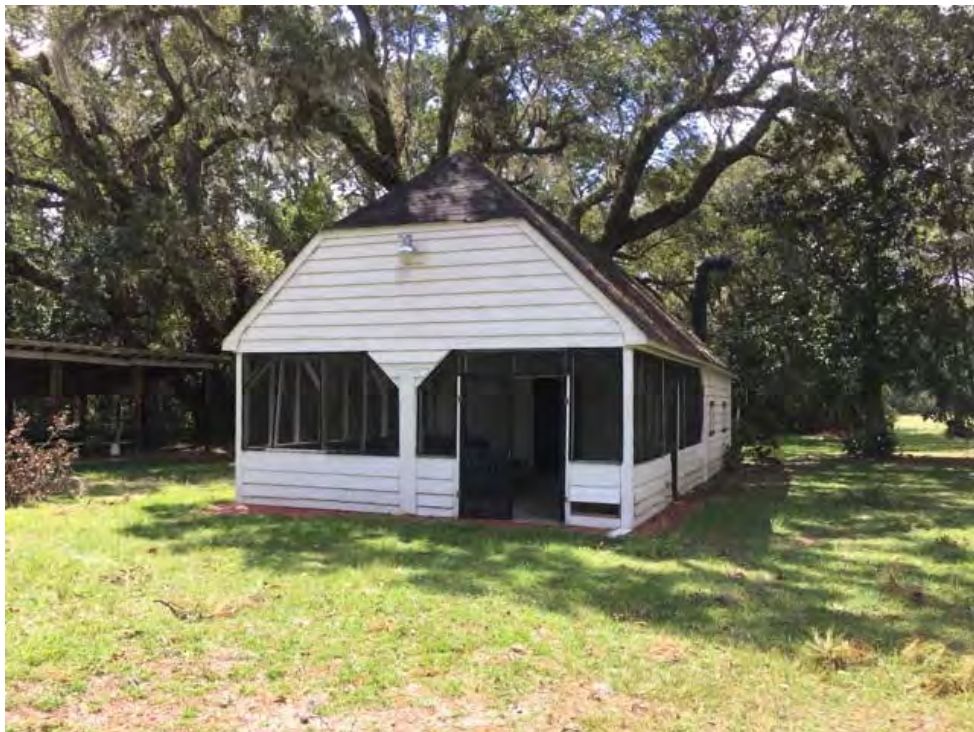
View of the partially screened storage building.
