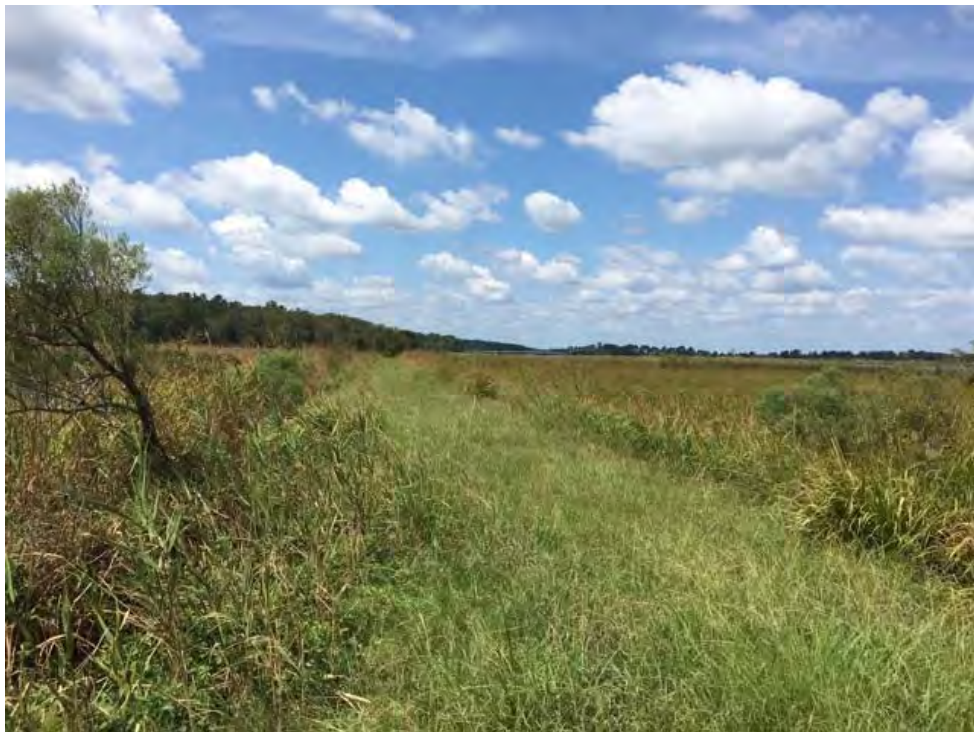
View of the dike paralleling the river.
