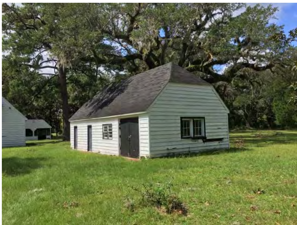
View of the enclosed storage building.
