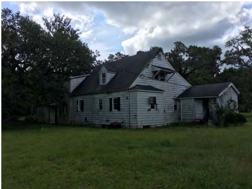
View of the old caretakers house that was converted to offices and is now in poor condition.
