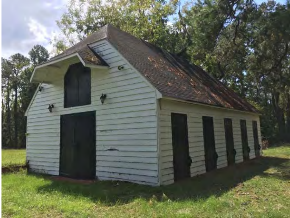
View of a stable looking building that is upfitted with old offices and not currently functional for recreational plantation use.
