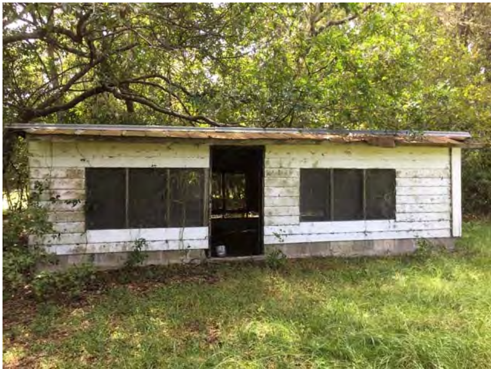
View of a miscellaneous shed located on the property.
