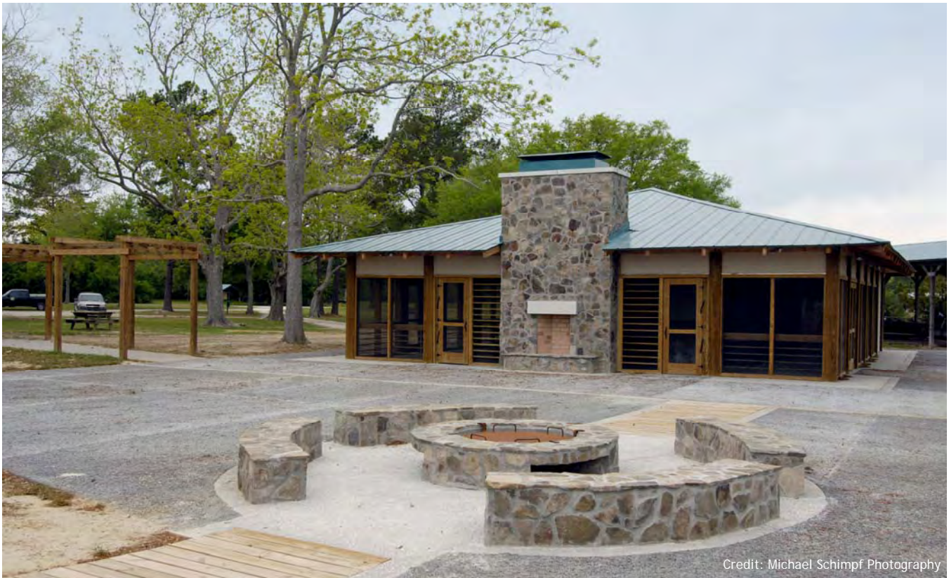
Bennett's Point's outdoor classroom, in the ACE Basin, uses pervious surfaces to improve water quality and manage stormwater drainage.
