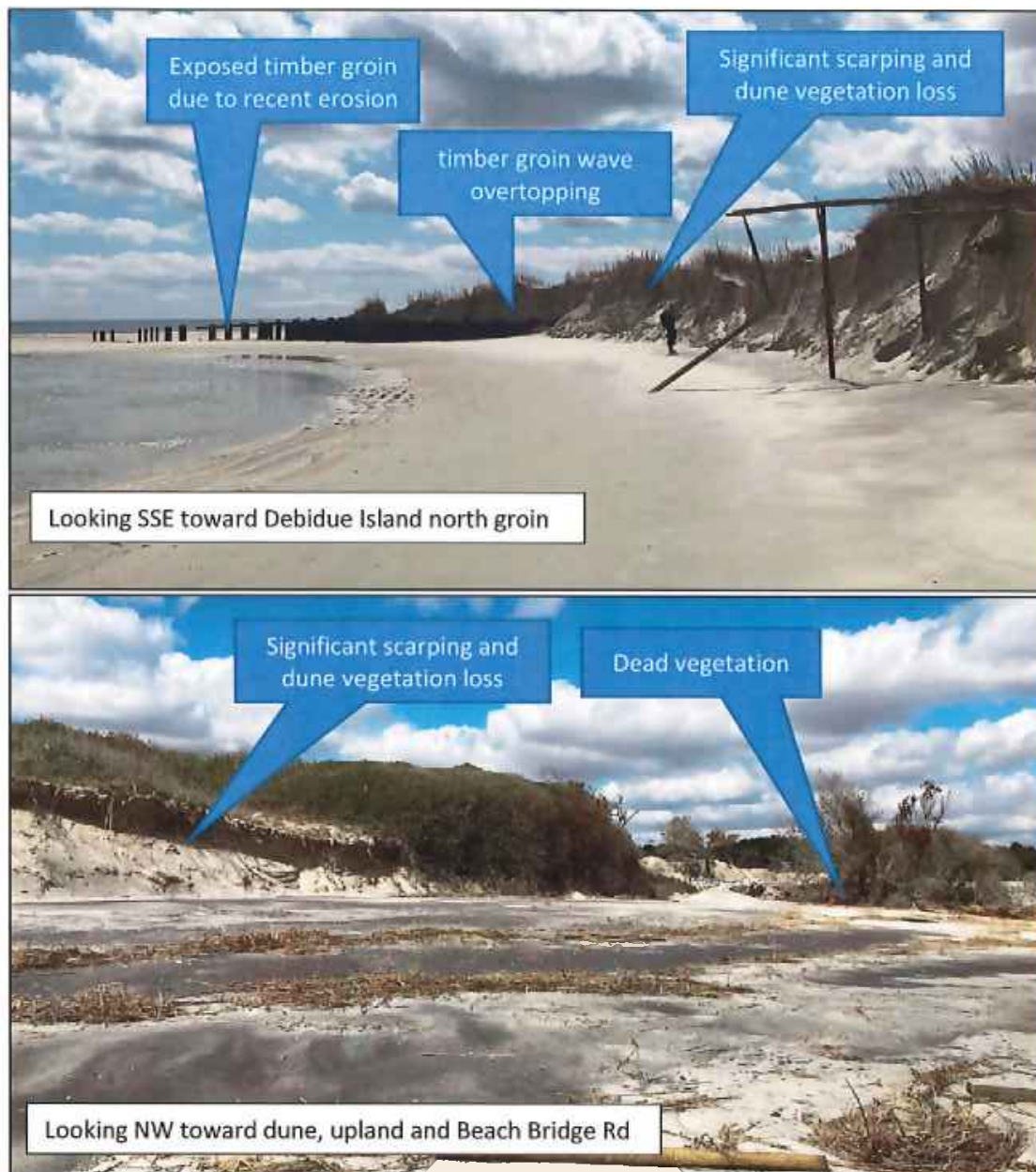
Figure 12: Site shoreline existing conditions along north end of Debidue Island (March 17, 2022). Note extreme scarping (8-10 ft high), vegetation loss, and exposed timber groin in marginal to poor condition.
