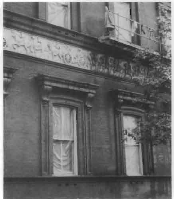
Figure 11. Removal of 100 years of grime from the brick and terra cotta facade of the Pension Building (now the National Building Museum), Washington, D.C., was accomplished by workmen on a swing stage using a chemical cleaning product. Note the polyethylene covering the windows to prevent damage. Also note the protective clothing for the workmen which hangs on the platform while not in use. Photograph: Christina Henry
