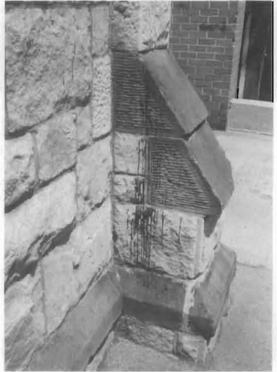
Figure 19. Efficient removal of tar splatters from limestone and sandstone may be facilitated initially by applying dry ice or carbon dioxide, but complete removal will probably require poulticing with an inorganic solvent.
