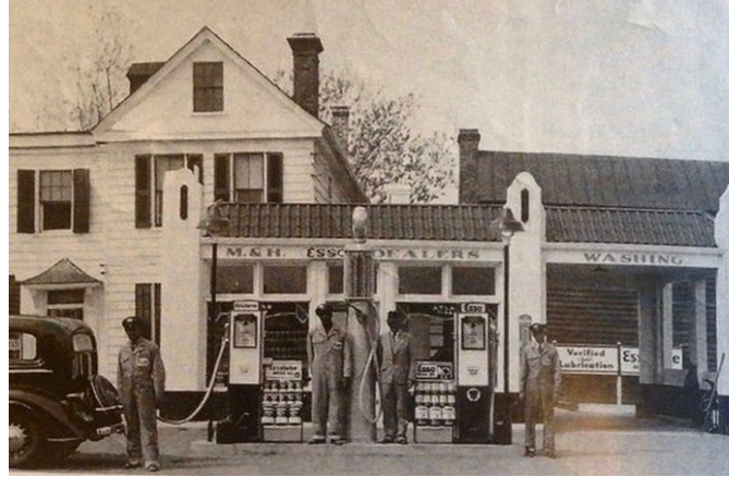
Photograph of Robert F. Morrison's Esso Station at 179 Coming Street, circa 1938
