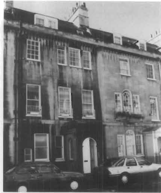
Figure 2. The building on the left is an obvious candidate for cleaning, as the heavy black crust may be concealing or contributing to deterioration of the stone. Despite its more recent cleaning, the stone facade of the house on the right exhibits the same distinctive, and hard-to-eliminate rainwater wash patterns under the eaves and window sills, as its unwashed neighbor.
