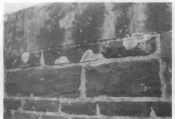
Figure 20. Plant growth such as lichens growing on a protected side of this limestone and granite parapet wall, can be damaging even to a relatively hard stone like granite because lichens secrete oxalic acid. Lichens can usually be removed, after soaking with water by scrubbing with a stiff natural bristle brush.
