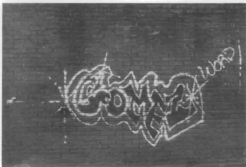
Figure 24. Spray-painted graffiti on this brick wall can be removed with paint remover, and in this case, probably will not require poulticing.
