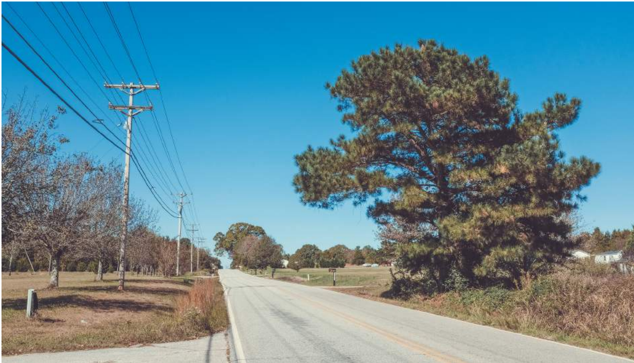
Rural road in the Five Forks area.
