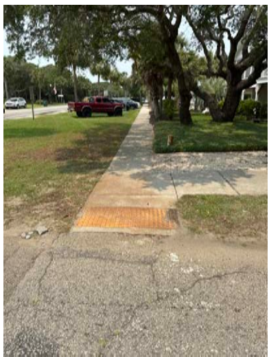
AT-GRADE SIDEWALK WITH TRUNCATED DOMES
