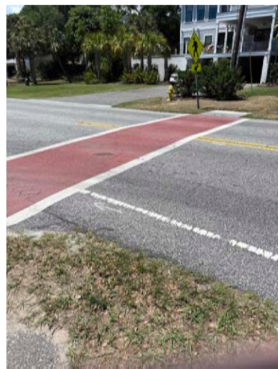
DELINEATED CROSSWALK WITH PEDESTRIAN CROSSING SIGN
