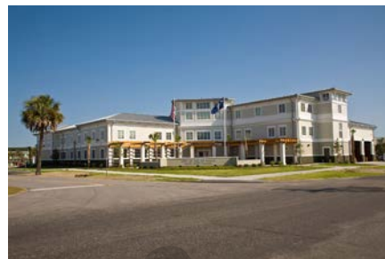
IOP Public Safety Building
