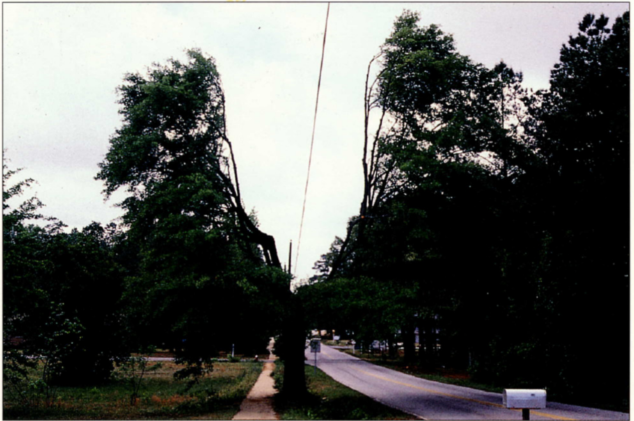
A proper top trim using the "V" trimming method.
