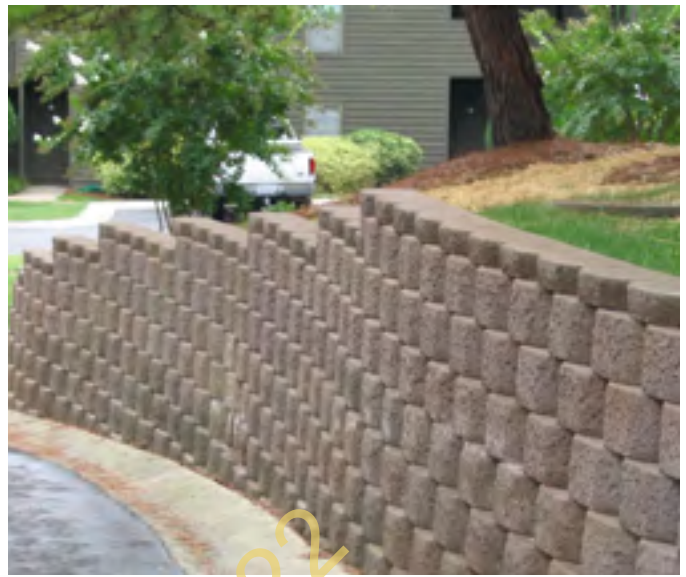
Illustration 6.3. Retaining Wall Example
