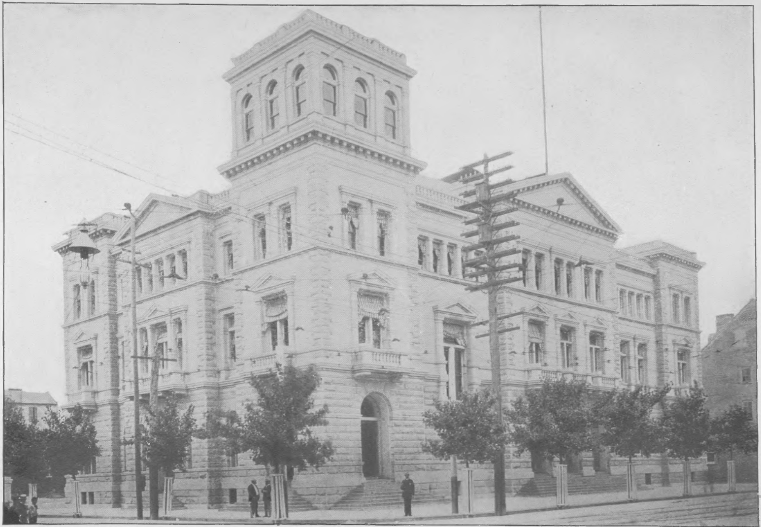
THE NEW POST OFFICE AND UNITED STATES COURT HOUSE.
