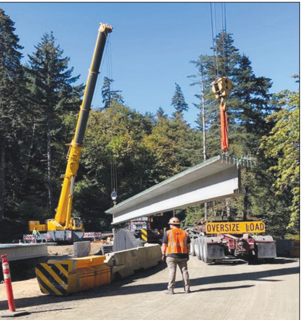
PHOTO CONTRIBUTED Workers replace the Little Luckiamute River bridge as part of the improvements to Mitchell Street and Black Rock Road near Falls City.
