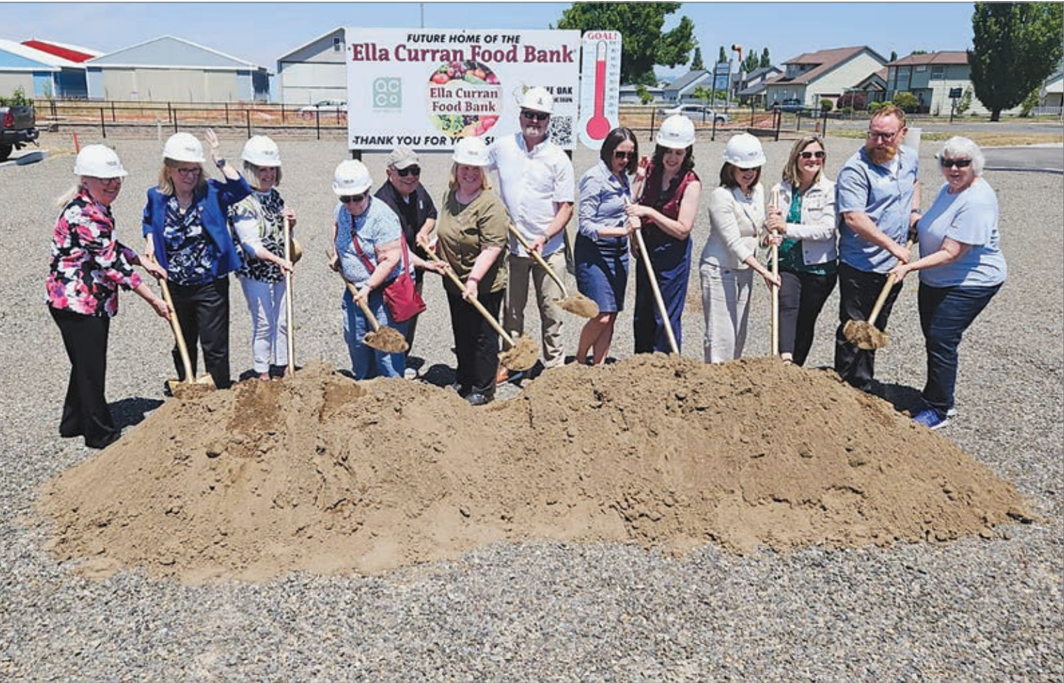
A large contingency of volunteers and dignitaries, both local and state, on July 7 dig the ceremonial first shovel of dirt at the Ella Curran Food Bank's new home at 750 Airport Road in Independence.
