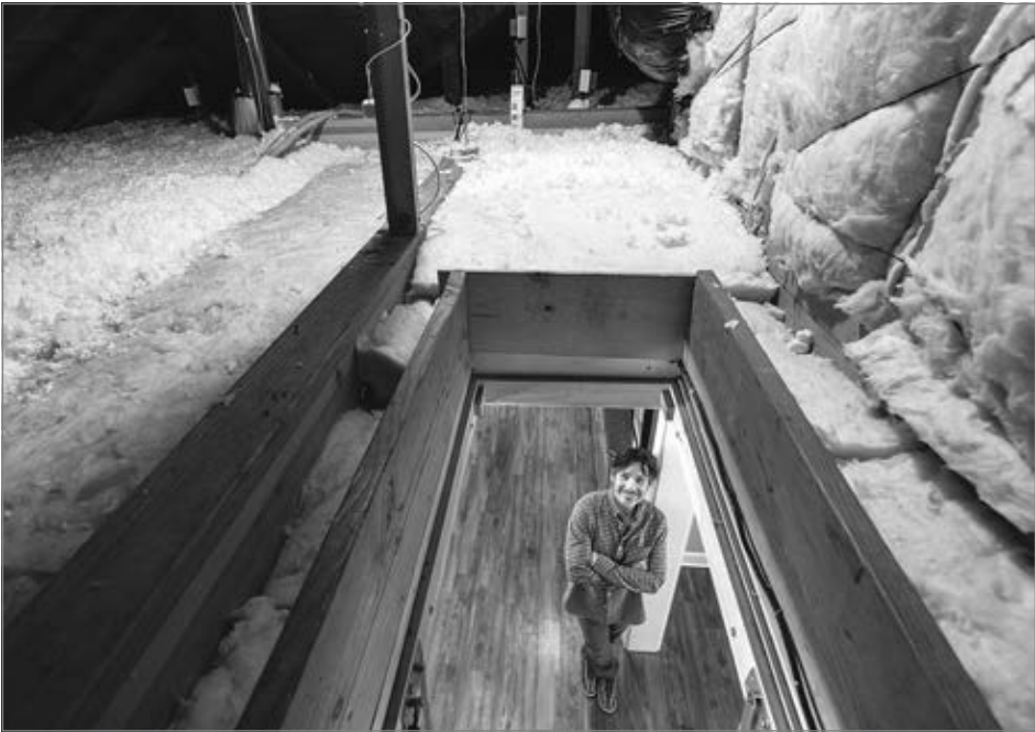
Garry Egan signed up for an Energy Trust program that replaced the insulation in his renovated home's attic.
