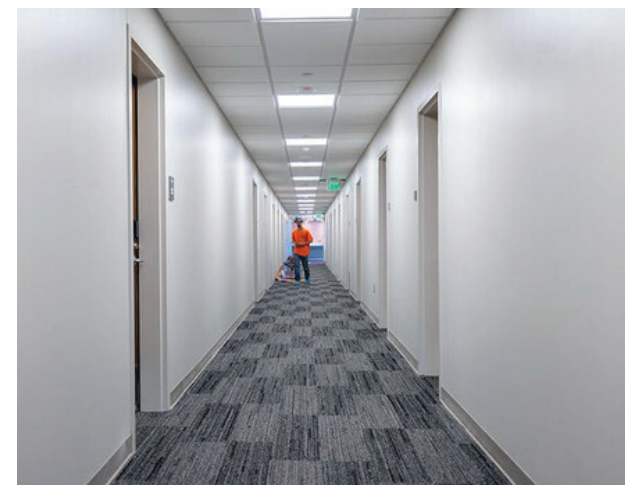
Interior McCasland Hall construction in June.
