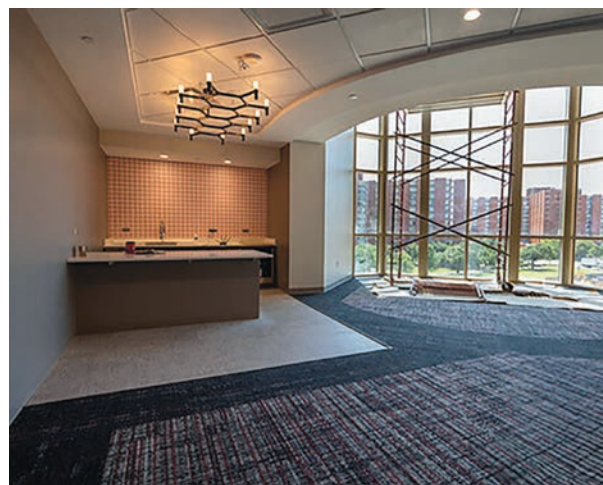
Interior McCasland Hall construction in June.
