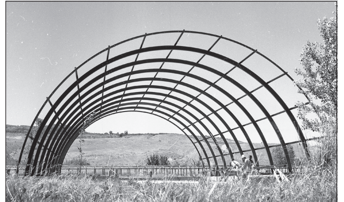
THE CHRONICLE New Quonset huts are constructed in 1965.
