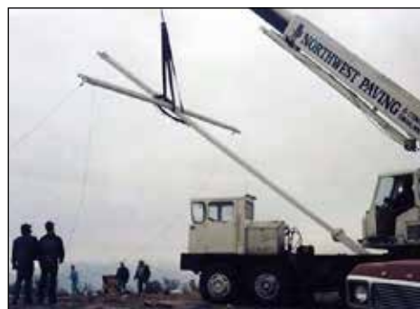
Erecting the cross in 1986.
