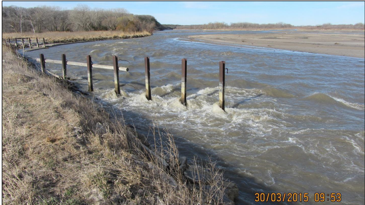
Figure 4.10 – Flow from south channel changing direction at the dike. (Corps of Engineers photo, 2015).
