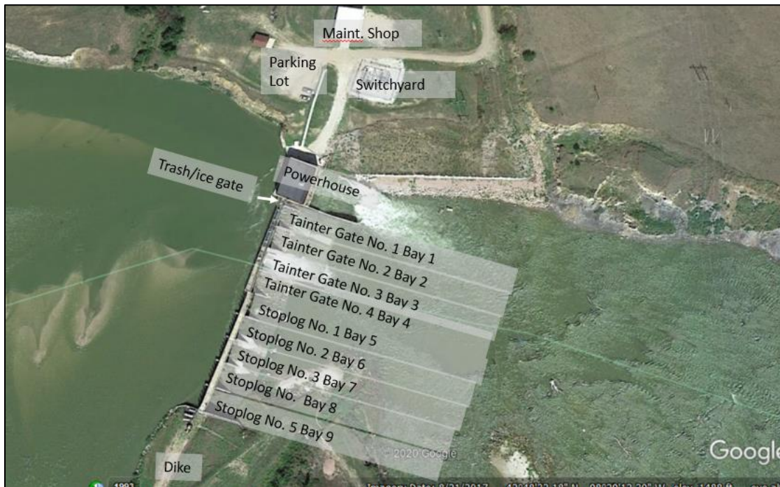
Figure 2.6 – Aerial view of Spillway, Powerhouse and other facilities – Source: Google Earth
