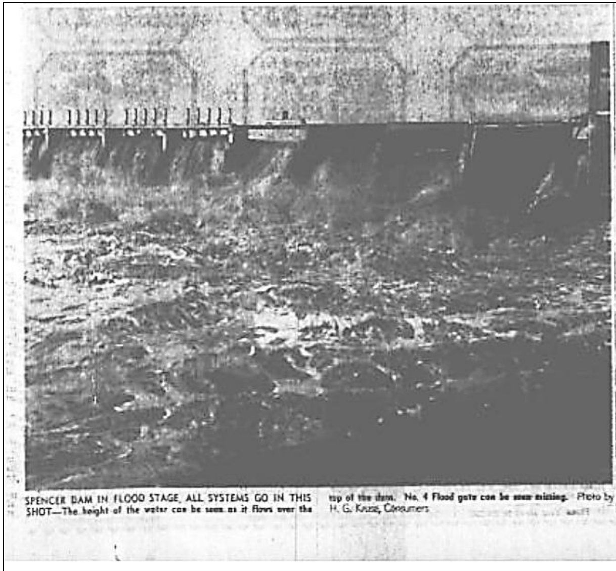
Figure 2.11 - Caption: "SPENCER DAM IN FLOOD STAGE, ALL SYSTEMS GO IN THIS SHOT" - The height of the water can be seen as it flows over the top of the dam. No. 4 flood gate can be seen missing. Photo credit Holt County Independent March 17, 1966, page 4. Research source: History Nebraska.
