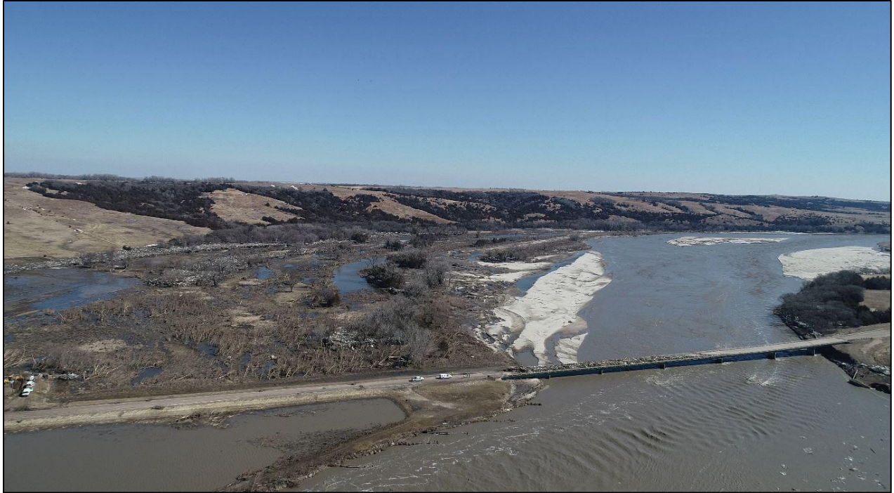
Figure 4.9 – Highway 11 Bridge and north approach looking downstream. Note the ice trapped between guardrails on the bridge and along the far-left bank (from NPPD video).
