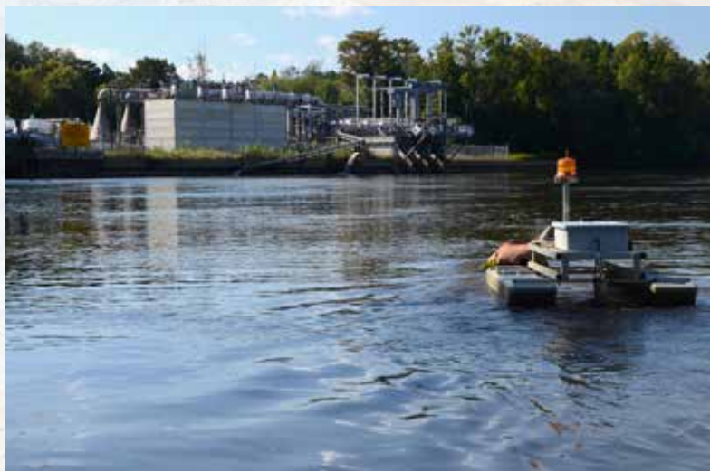
The U.S. Army Corps of Engineers dissolved oxygen injection system operates on the banks of the Savannah River. The facility injects oxygen into the river to support habitat for aquatic wildlife, including federally protected fish species. The Savannah River TMDL for dissolved oxygen forced more than 20 municipal and industrial dischargers to work to reduce their impact on the river and prompted the construction of this facility to mitigate impacts from the deepening of the Savannah Harbor.
