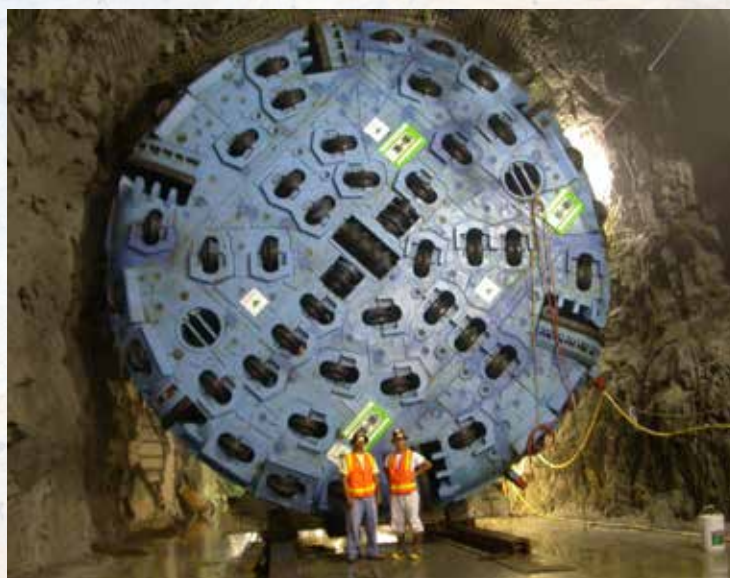
Upper Chattahoochee Riverkeeper's (now Chattahoochee Riverkeeper) Clean Water Act lawsuit against the City of Atlanta forced the city to comply with the federal law and initiated $2 billion in sewer infrastructure projects including an 8.5-mile tunnel capable of storing 177 million gallons of untreated sewage. The tunnel dramatically reduced combined sewer overflows that plagued the city's sewer systems during rain events and polluted the Chattahoochee with fecal bacteria.
