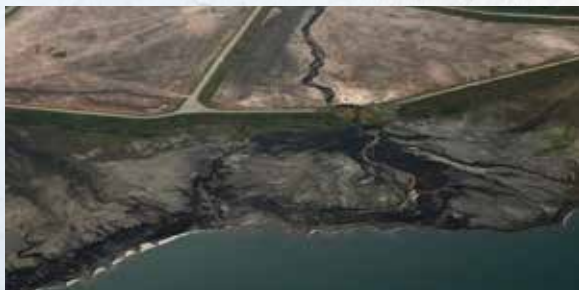
Georgia Power intends to leave tons of toxic coal ash in unlined pits at its power plants along the Chattahoochee and Ocmulgee rivers. Monitoring reports show coal ash pollutants in groundwater surrounding these pits.
