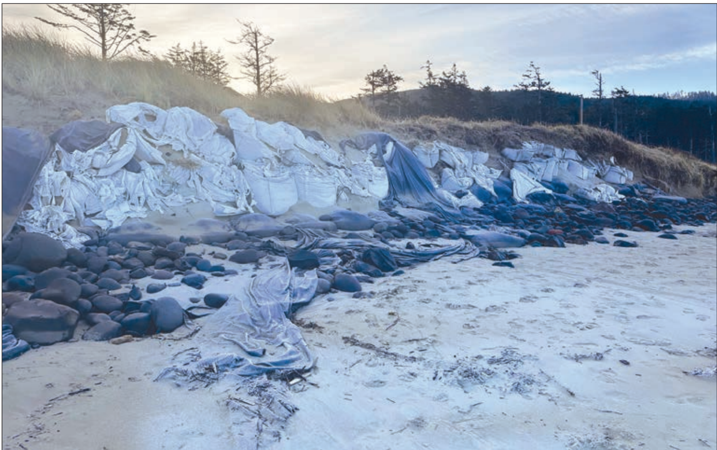
The section of the manmade dune at Cape Lookout State Park that has experienced the most sloughing because of wave and storm action and that will be repaired as part of the coming work.
