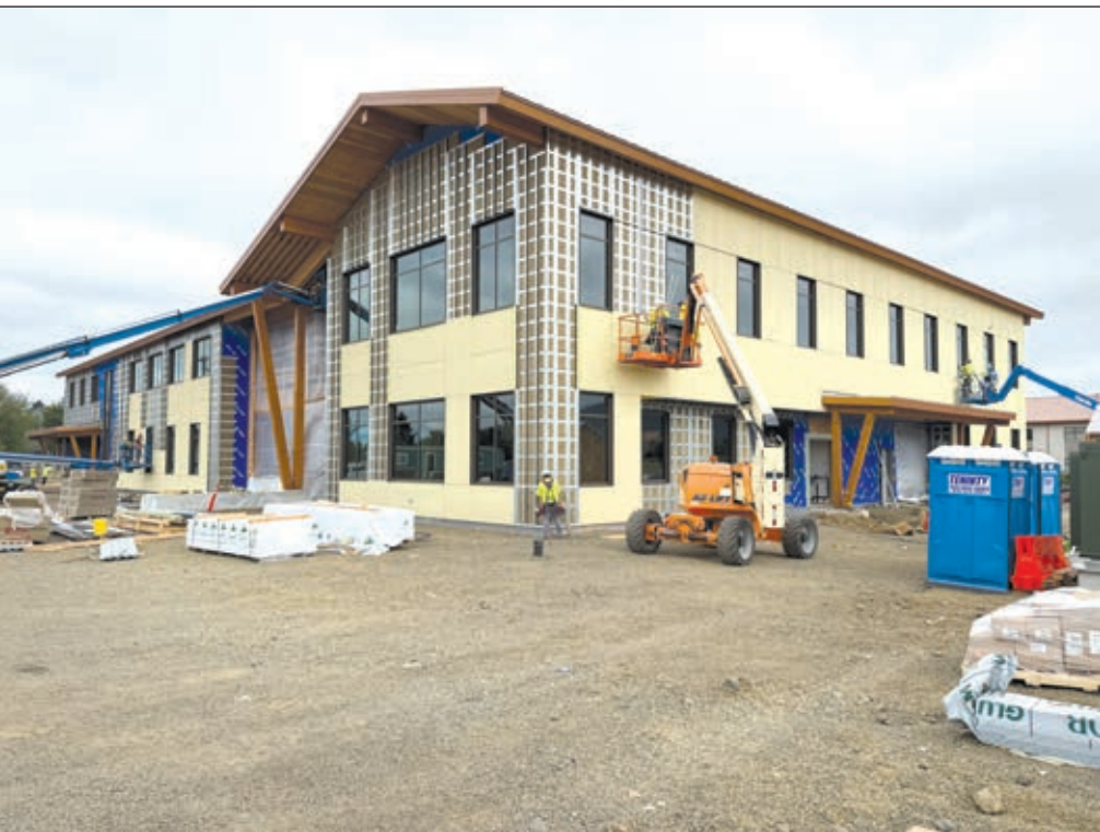
Tiling being installed on the new healthcare education building’s exterior that will be painted to match the main building.
