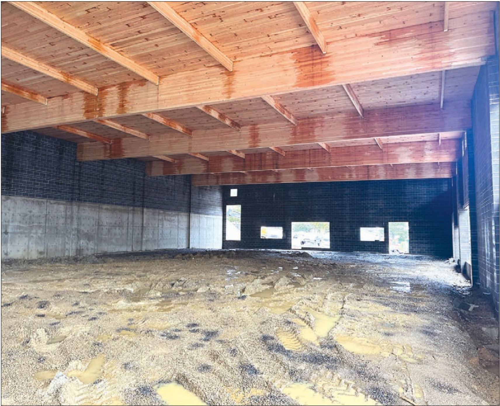
The interior of the new pool building at the North Coast Recreation District featuring a mass timber roof.
