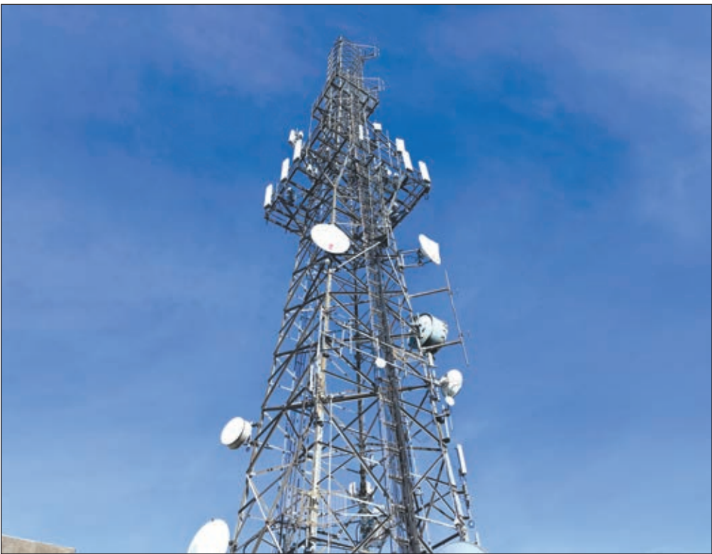
PHOTO BY WILL CHAPPELL The tower on top of Cape Meares that hosts transmitters for the county's emergency radio system, as well as a plethora of other broadcast, cellular and amateur and professional radio equipment. In addition to sometimes competing for frequencies, the large number of loose cables left by past users cause literal noise on radios as they move in the wind.
