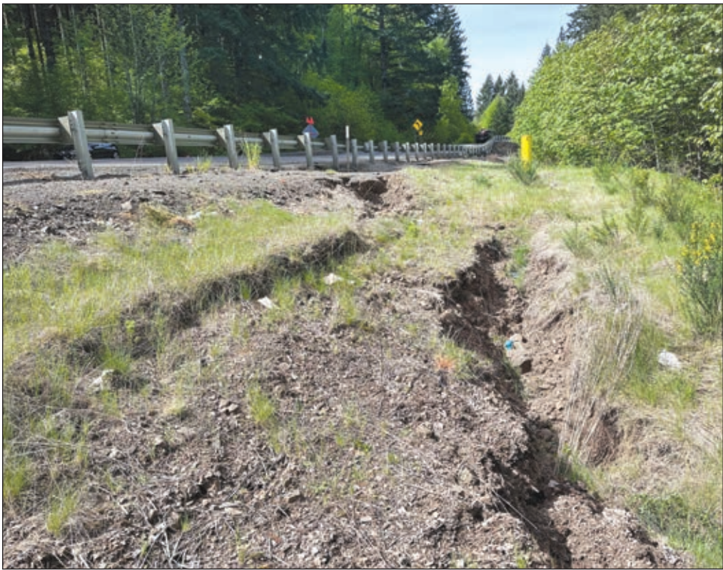
The downhill side of the road at the slide site is fissured and the layers of pavement, as well as wood chips, used in various repairs over the years are clearly visible.
