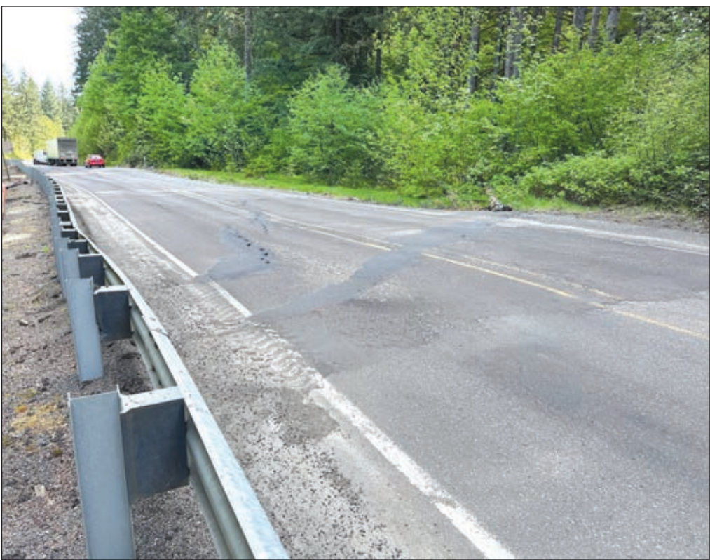
Cracks and patches abound on the roadway in the areas affected by slides.
