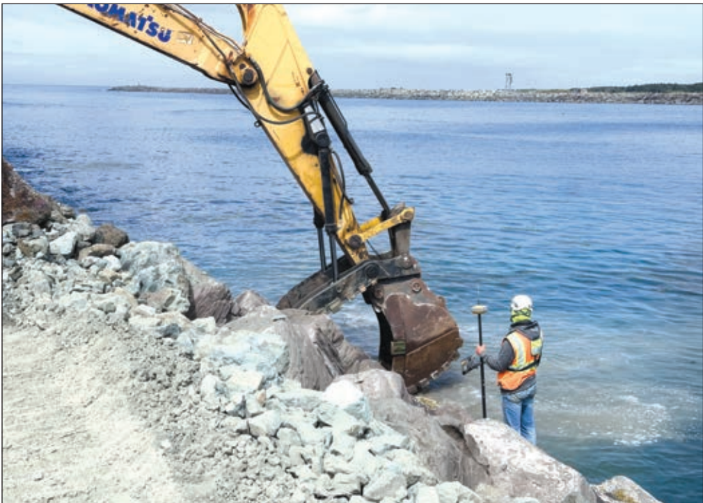
PHOTO BY WILL CHAPPELL The stone placement team's spotter inspects the excavator's placement of a stone, prepared to log its location with a GPS beacon.
