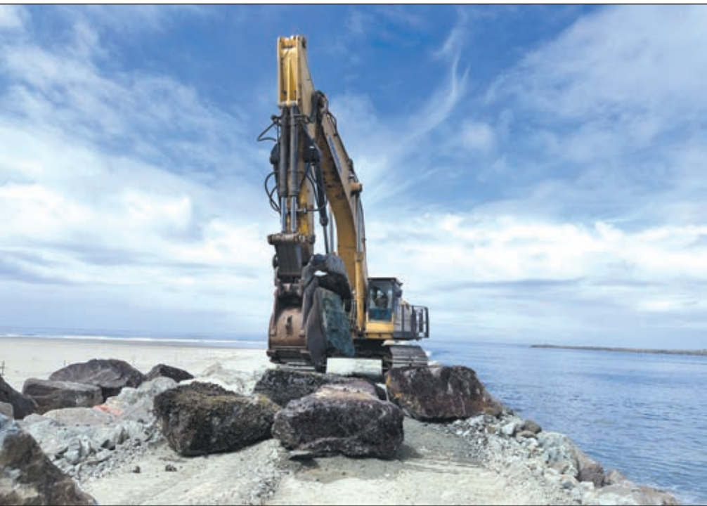
PHOTO BY WILL CHAPPELL The excavator moves a legacy stone from the jetty's original construction. Some of these stones are being moved to make place for new stones, but they will all end up back in the jetty, usually near their original location.
