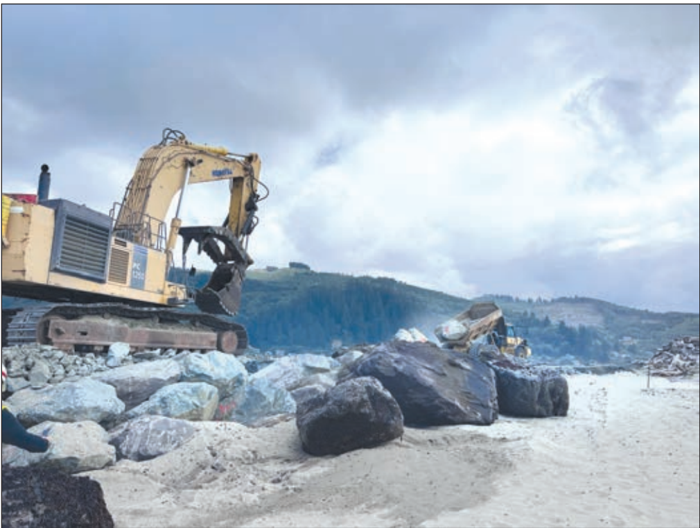
PHOTO BY WILL CHAPPELL A transport truck dumps three stones on top of the jetty for the waiting excavator to place.
