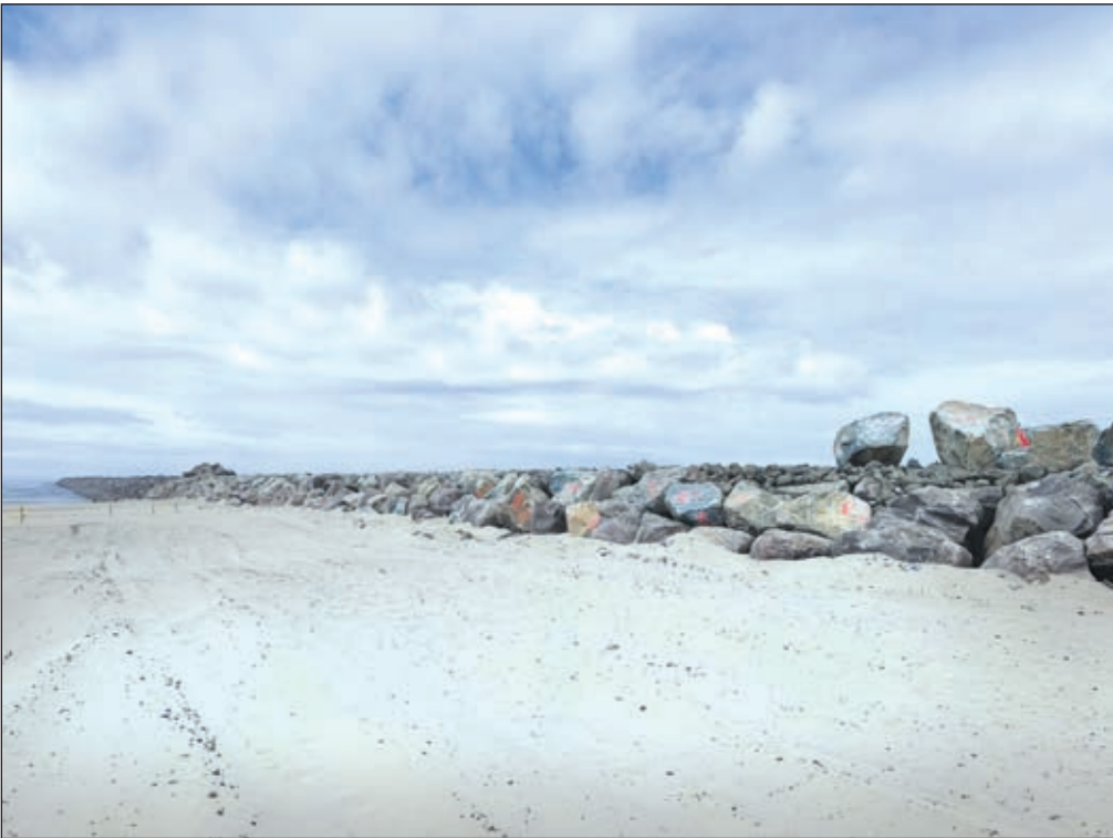
PHOTO BY WILL CHAPPELL The 600-foot section at the trunk of the jetty that has already been repaired.
