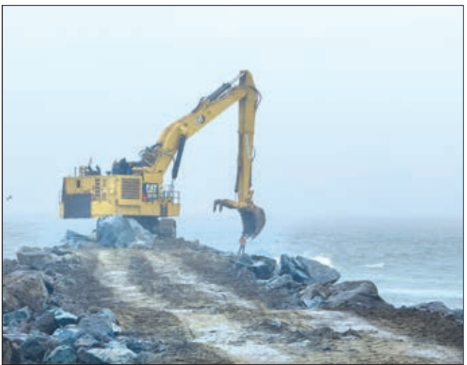
A crew at work placing stones near the head of the south jetty.
