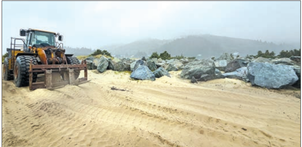
A front-end loader at the secondary staging area near the jetty's trunk with stockpiled stones.
