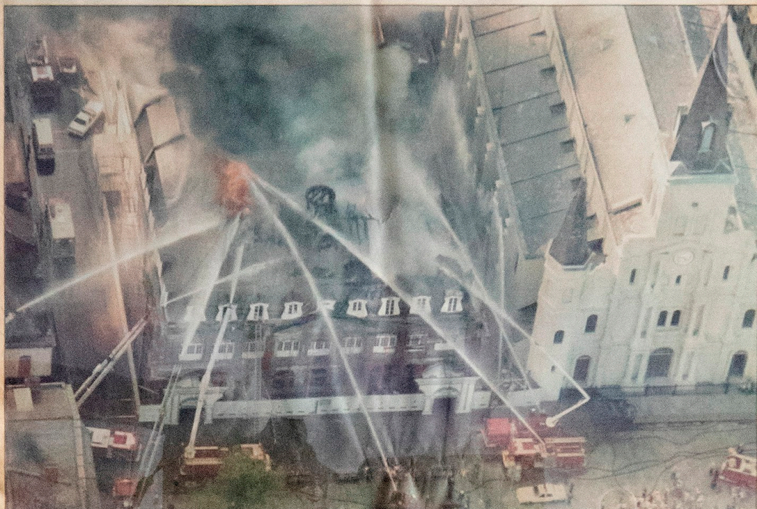
With scores of firefighters on the scene, aerial hoses spray water onto the Cabildo's roof as the seven-alarm blaze burns out of control.
