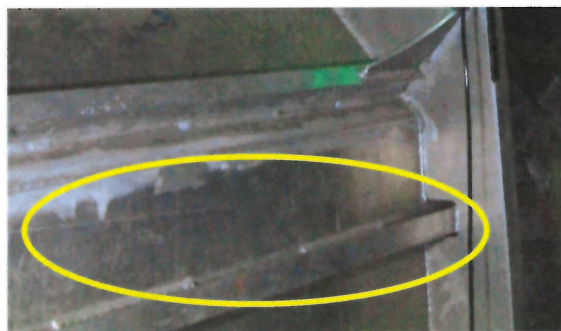
Figure 4: Stiffeners Below Haunch Knuckle
