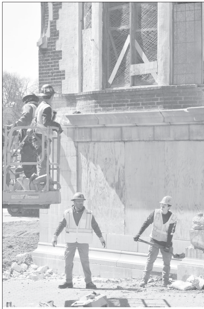
Workers prepare the Flanagan site for the building's demolition. Richard Rosentreter photo
