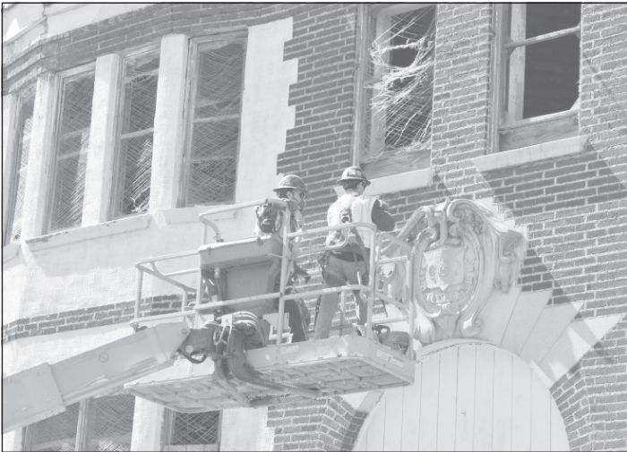
Days before the Flanagan’s demolition started, workers from Binghamton-based Gorick Construction Co. planned an attempt to salvage several historic features of the building, such as the stone carving at the front of the structure. Richard Rosentreter photo
