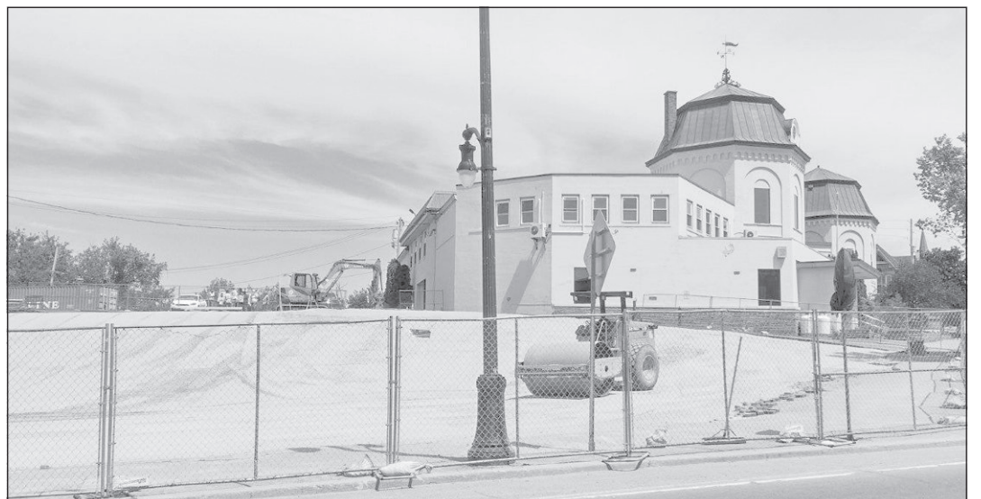
The former site of the Flanagan hotel as seen in late May 2026 after its demolition. Richard Rosentreter photo
