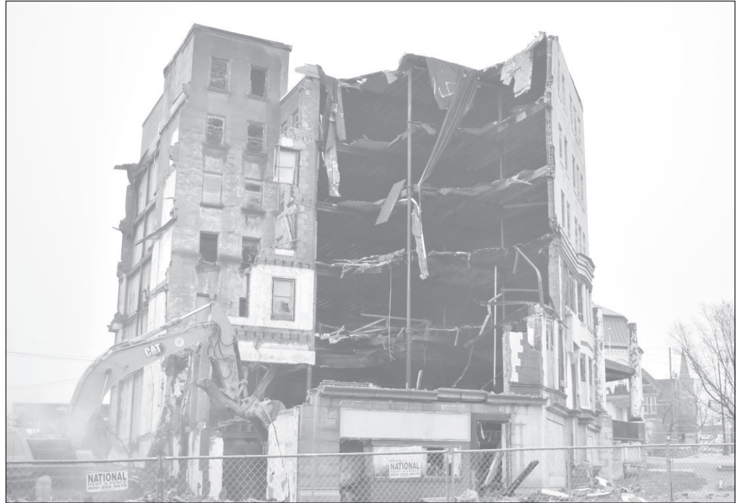
By the third day of the demolition, a large portion of the Flanagan had been reduced to rubble. Richard Rosentreter photo
