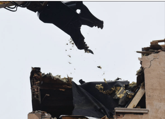
The heavy equipment used in the demolition looks more like a dinosaur as it takes the first chunks from the Flanagan on the first day of the project. Richard Rosentreter photo
