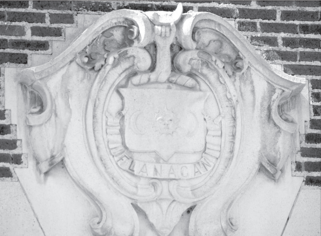
An engraved stone piece that was above the main entrance of the Flanagan. It is not known if the demolition crews were able to salvage it. Richard Rosentreter photo
