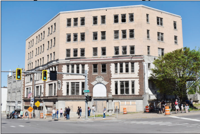
The former Flanagan hotel at the corner of Elm and Main streets in Malone. Richard Rosentreter photo
