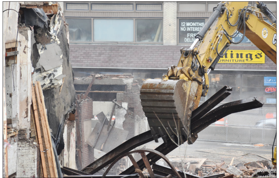
Demolition underway at the Flanagan in Malone. Richard Rosentreter photo.
