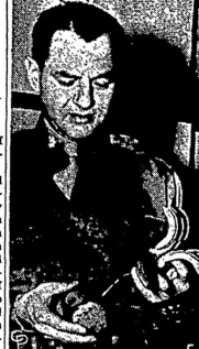
NAZI 'BUTTERFLY' —A German "butterfly" anti-personnel bomb is examined by Maj. Martin L. Ehrmann, New York, Commandant of the Bomb Disposal school at the Aberdeen, Md., Proving Ground. The bombs are dropped from planes in clusters. He holds in his right hand the cap containing the explosive charge, and in his left the opened "wings." When the bomb is released, the wings act like a parachute and slow down its descent. Army photo.
