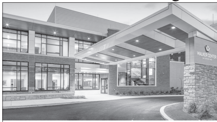
The Walker Center for Cancer Care at Samaritan Medical Center in Watertown. Contributed.
