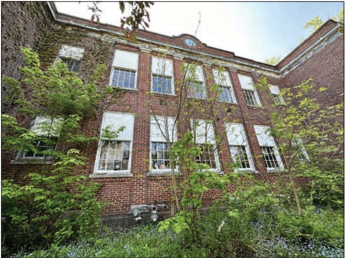
Naturally Lewis is seeking ways to reuse the former Lyons Falls Elementary.
