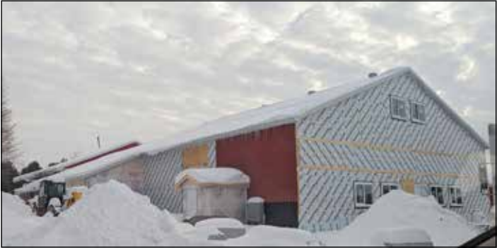
Red Barn Meats expansion project underway in January. Contributed.
