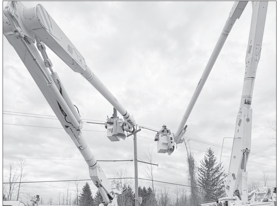
supporting fellow utilities and the significant impact of mination of their workforce, Crews repair a line in Brockport following Winter Storm Iona. Contributed
