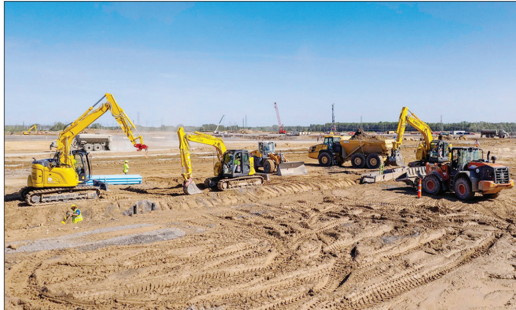
In early July, Micron celebrated the first concrete pour milestone at its Clay site, which occurred more than one quarter ahead of the original plan and marked the transition from site preparation to vertical construction. Micron plans to invest up to $3 billion to develop the domestic semiconductor supply chain ecosystem in support of its U.S. manufacturing footprint. Micron
