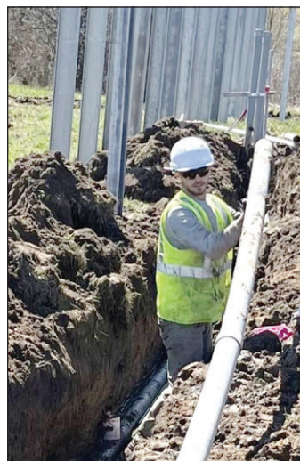
Luke Frederick of IBEW Local 910 works on a solar farm project. Local 910 photo
