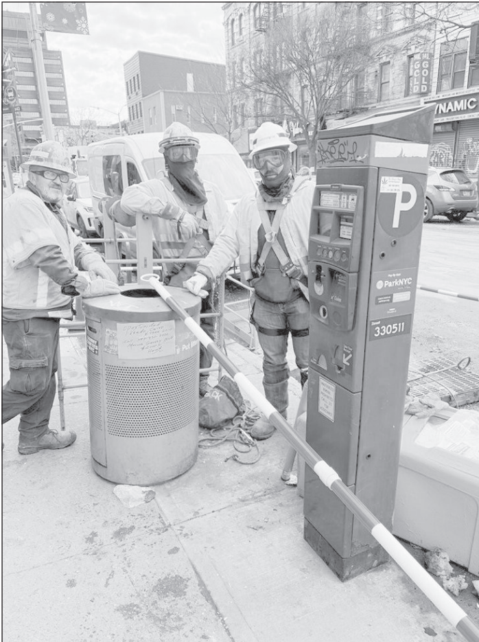
Underground line mechanics from National Grid in Brooklyn assisting Con Edison as they recover from a multi-day outage in early March. Contributed.
