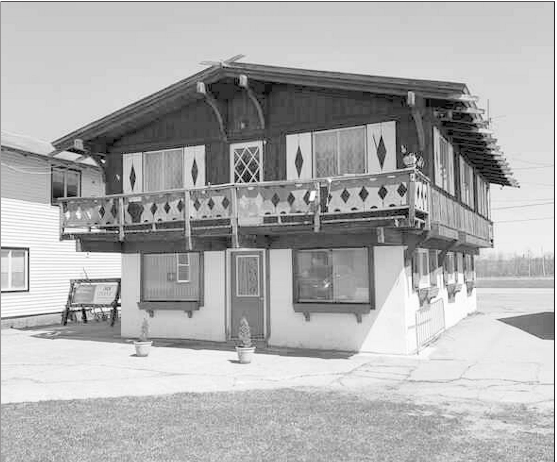
The owners of Snow Ridge Ski Resort will use the grant from the first round of the Lewis County Development Corporation's Vacant Property Revitalization Program to transform the top floor of this Alpine-styled building in Turin into a short term apartment rental space. Photo provided
