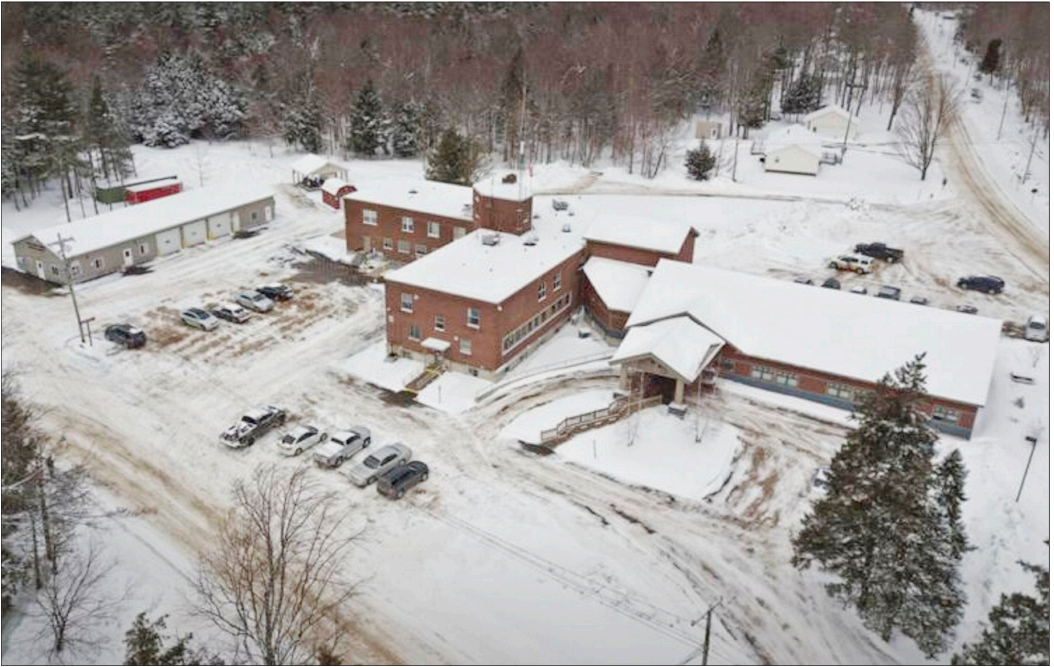
Clifton-Fine Hospital, a 20-bed critical access center in Star Lake, is planning extensive renovations to its emergency department as it prepares to convert to a Rural Emergency Hospital, Christopher Lenney/Watertown Daily Times
