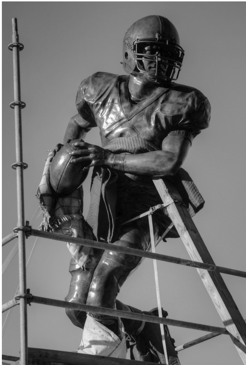
Installation of the football player statue outside Jerry Richardson Stadium in January 2013. | Niner Times File Photo
