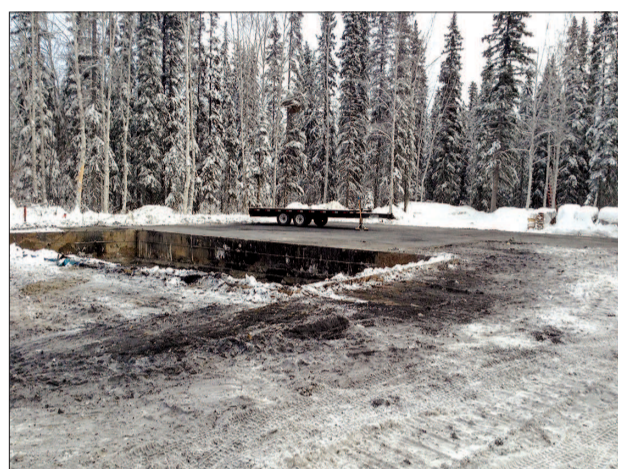
The remains of 2180 Shale Court, property owned by Ron and Jane Hunt, after a fire Jan. 8. PHOTO COURTESY RON HUNT
