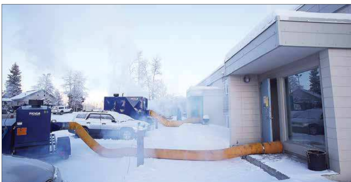
Portable heater hoses run into Walsh Hall at the University of Alaska Fairbanks on Monday after a steam line broke, cutting off heat and hot water to several buildings. ERIC ENGMAN/NEWS-MINER
