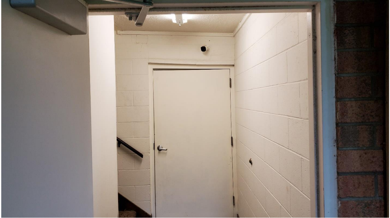
Out of Plumb Door Jamb, Entry Door Along East-West Wall Line – Facing North
